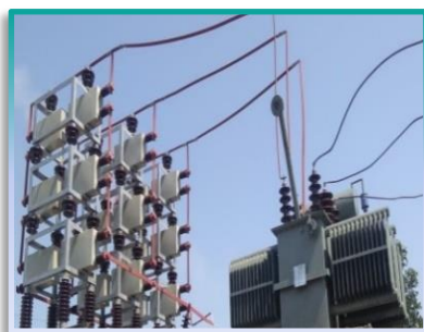
HT Passive Harmonic Filters
