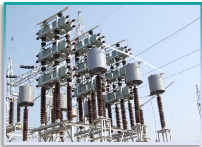
HT Capacitor banks of voltage levels from 3.3 kV to 132 kV
