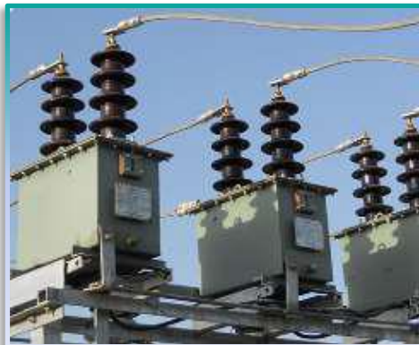
MV Current and Voltage Transformer upto 33 kV
