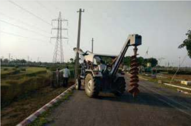
Fixing of electric poles at Florence Town, Jaipur
