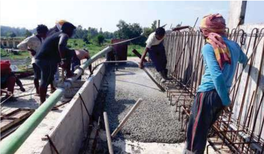
Bridge under Construction at Florence City, Pathankot
