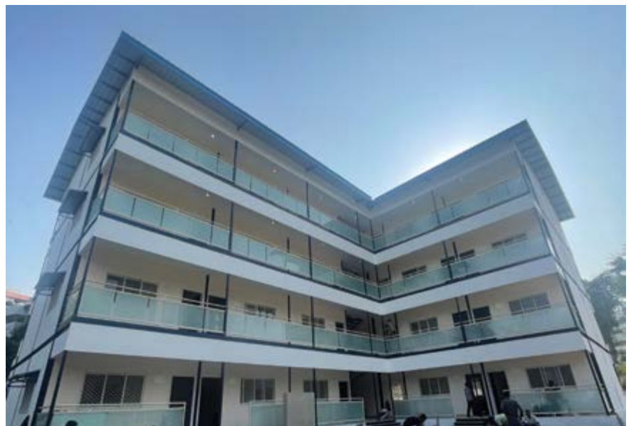
Construction of Hostel for Veer Naris (War Widows) at Mankhurd
