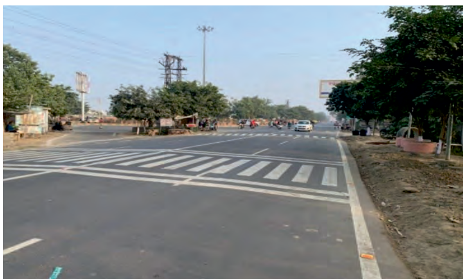
Road restoration and repair works Udaipur, Rajasthan.
