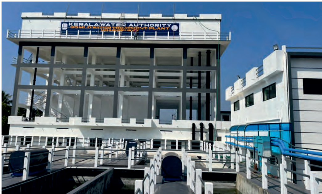
Water Treatment Plant at Chengannur Municipality, Kerala
