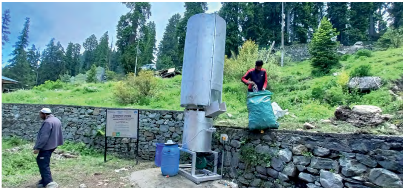
Gasifier at Gulmarg , Srinagar Gondola site for plastic waste management
