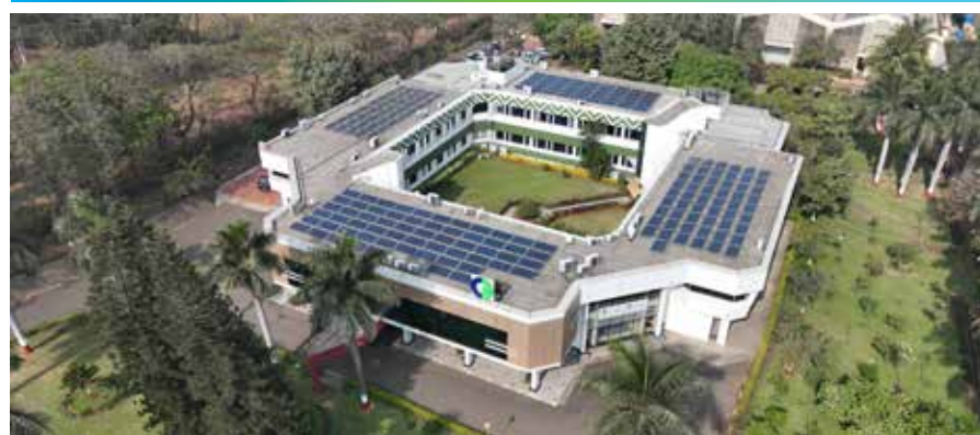
Switchgear Complex Admin Building, Nashik
