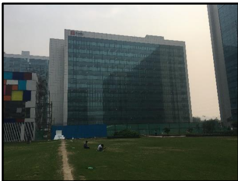
View of Tower 9
