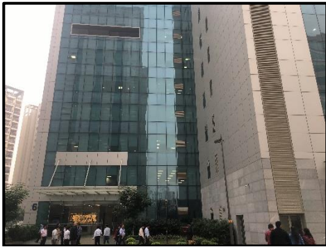
View of Tower 6
