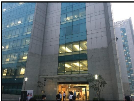
View of Tower 5
