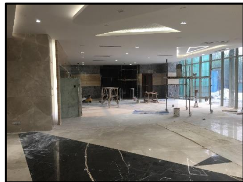
Internal view of Tower 8
