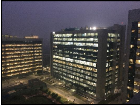
View of Tower 1
