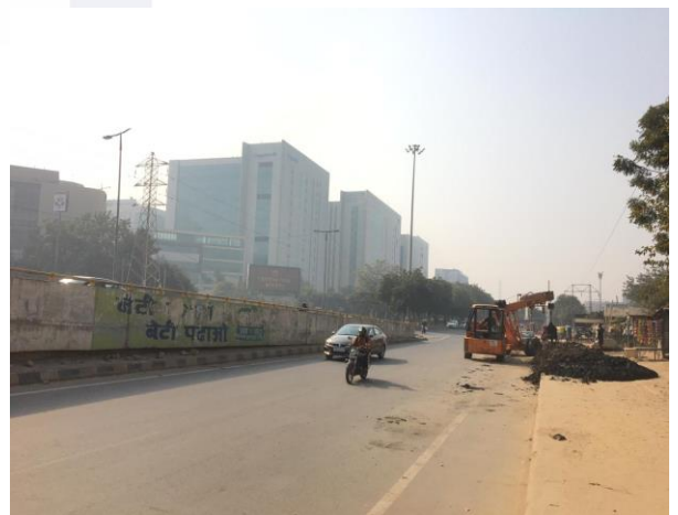
View of the Access Road
