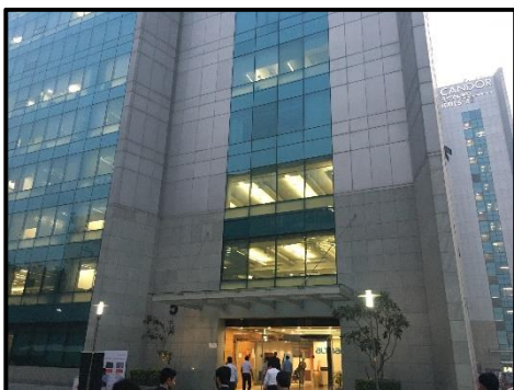
View of Tower 5
