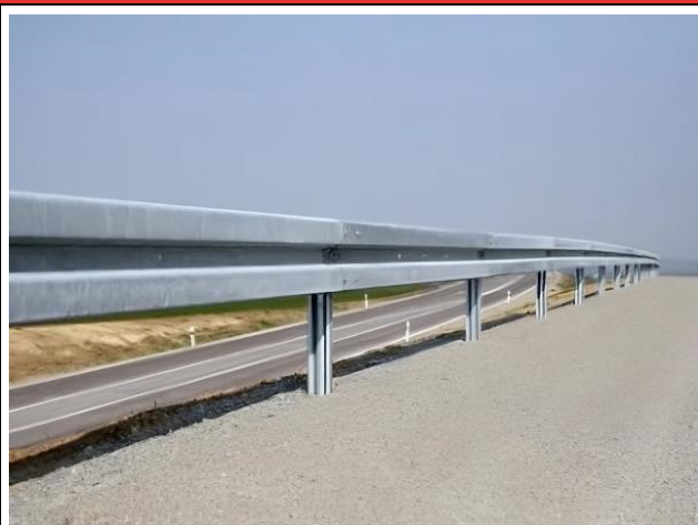
METAL BEAM CRASH BARRIER
