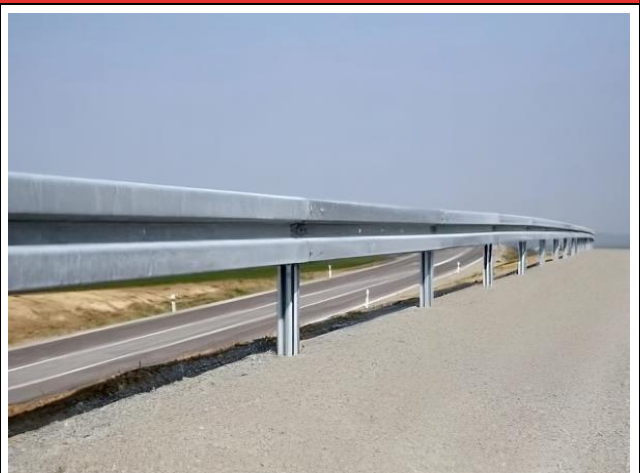
METAL BEAM CRASH BARRIER
