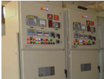
Indoor MV Switchgears upto 33 kV
