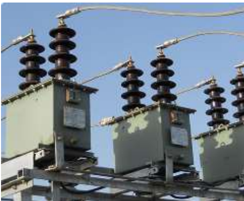
MV Current and Voltage Transformer upto 33 kV
