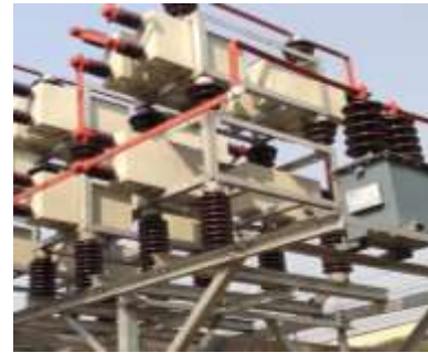
HT Capacitor banks of voltage levels from 3.3 kV to 132 kV
