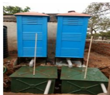
FRP Toilet With Bio-Digester Tank
