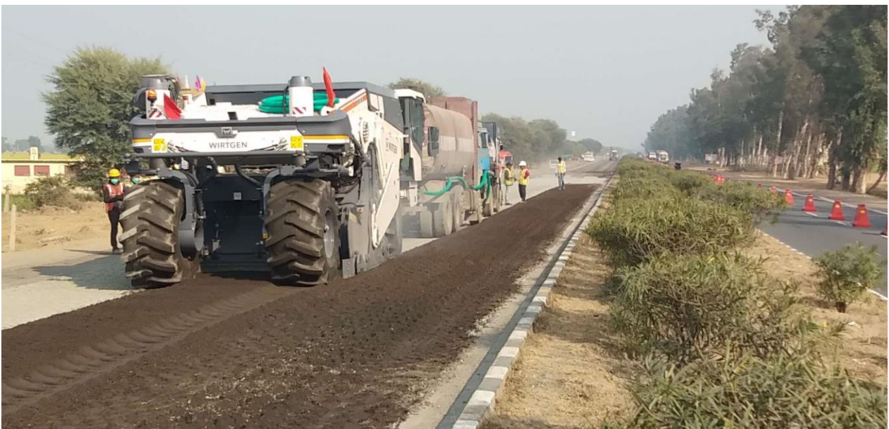
Figure 8. Cold-In-Place Recycling:
