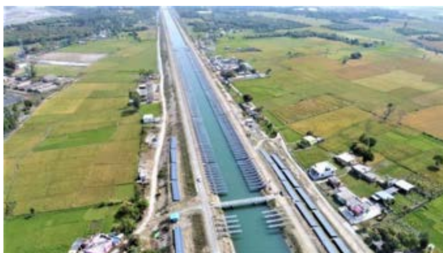
Canal top solar power plant on 35-meter-wide Yamuna Power Channel in Uttarakhand installed by our Company using suspension rope technology
