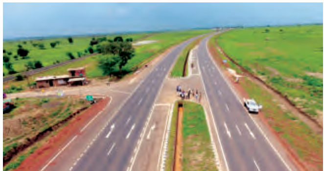
Shivpuri-Guna Four Lane Highway project
