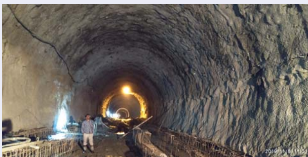
Tunneling work for the Jiribam-Tupul rail line project
