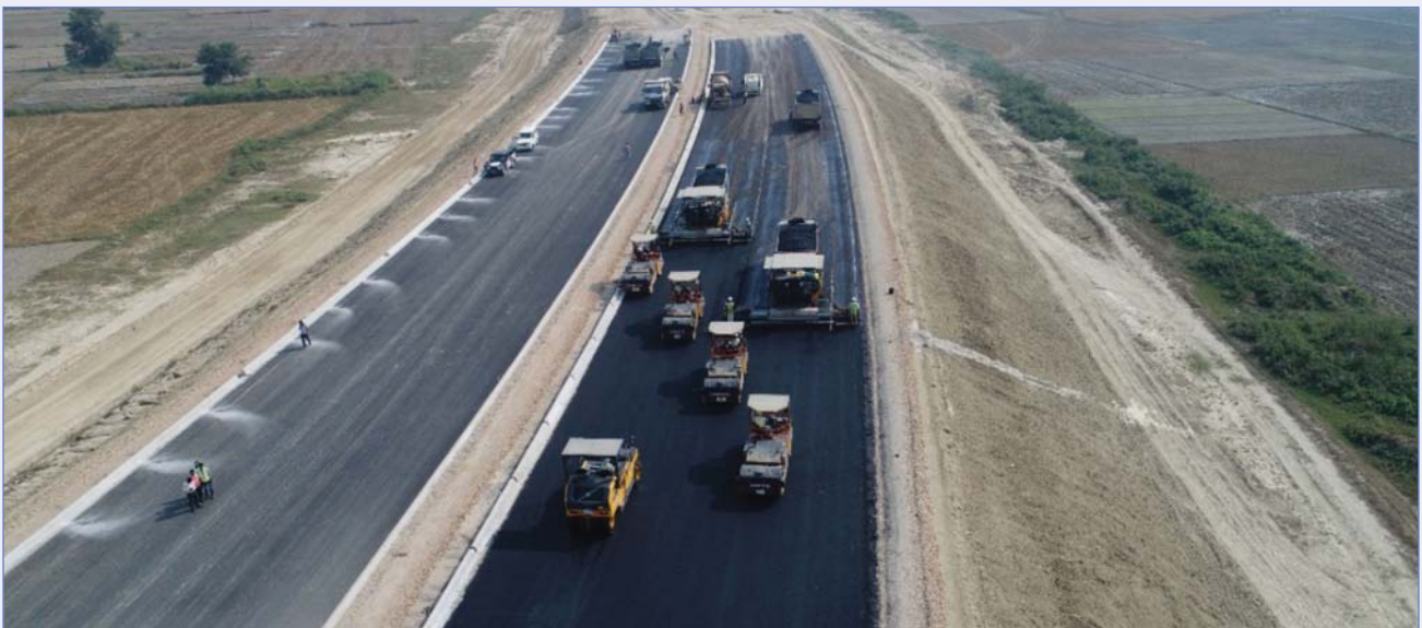
PMC-cum-External Technical Auditor for Purvanchal Expressway
