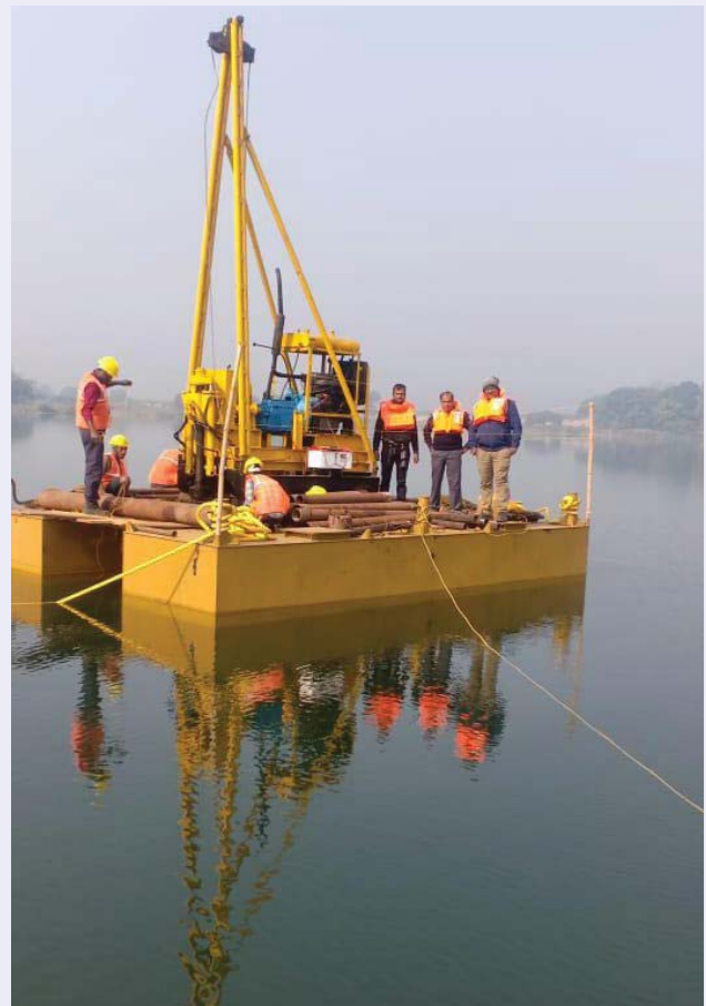
Drilling in progress for Obra Dam, East Coast Railway
