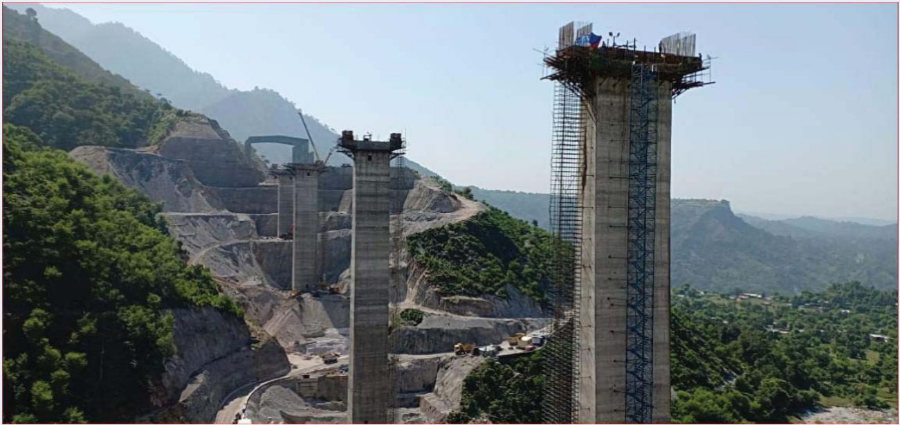
Bridge construction under the Udhampur-Srinagar-Baramulla Rail Link project
