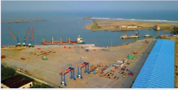
Independent Engineer Services for developing Multipurpose Berth at Paradip Port, Odisha
