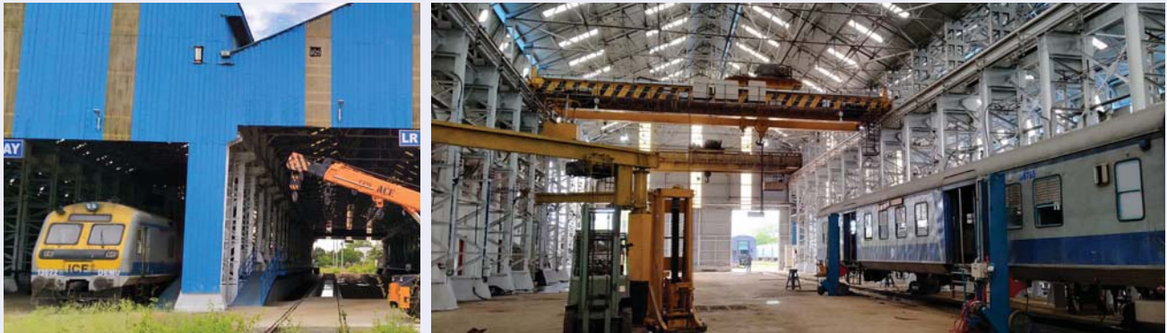
Setting up of DEMU car shed at Lumding, Assam
