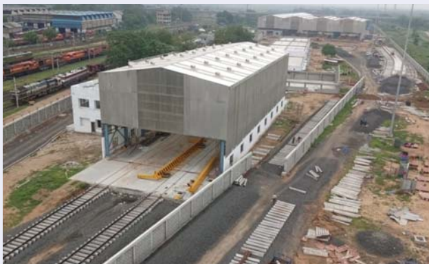
Construction of CPOH and DMC workshop at Vatva, Ahmedabad
