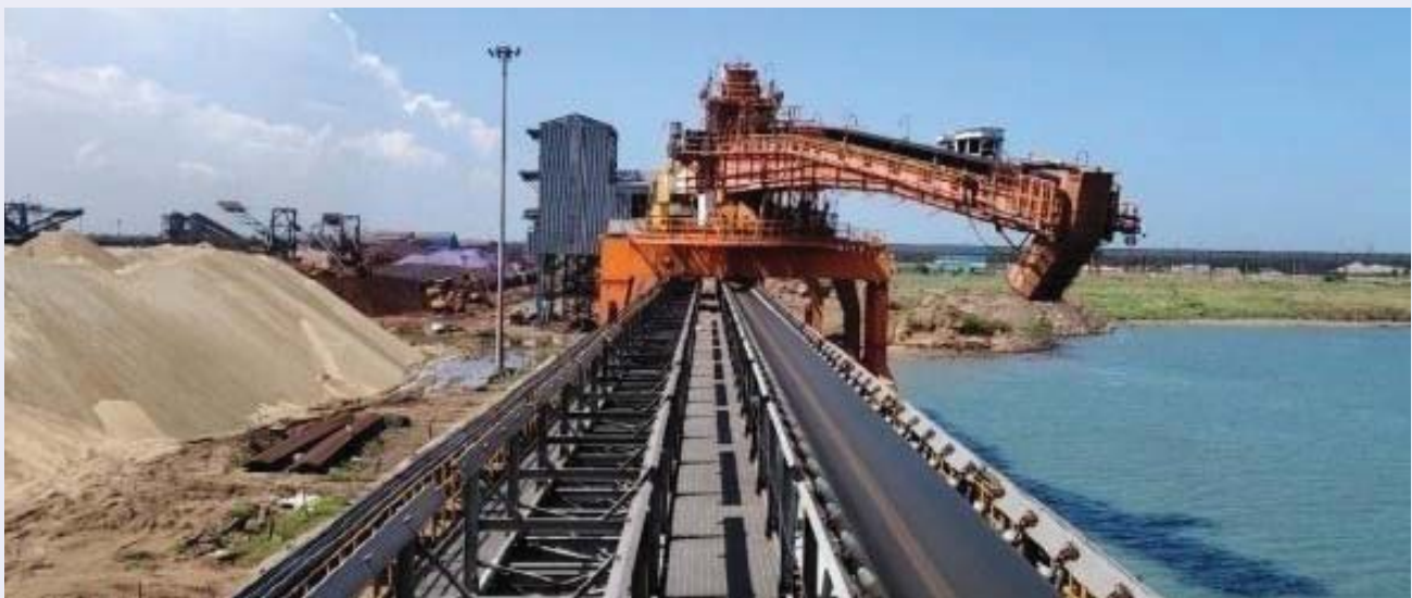
Iron Ore Export berth with mechanical handling facilities ready for commissioning
