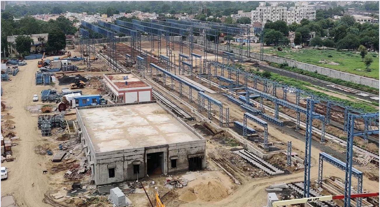
Construction of flash-butt welding plant at Sabarmati, Gujarat
