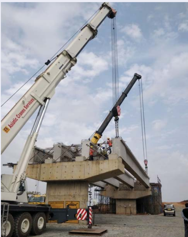
Girder launching along Baharagora to Singhara section in Odisha
