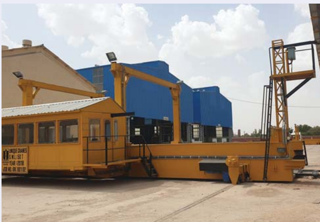
POH facilities for BCN and BLC wagons at North Western Railway Workshop, Bikaner
