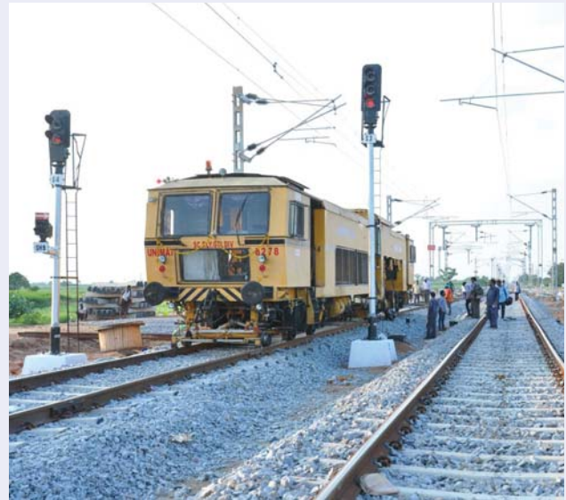
Doubling of railway track at Gooty-Dharmavaram in Andhra Pradesh
