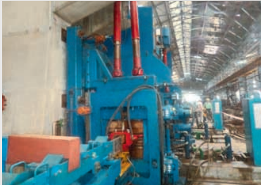
Newly erected vertical stand of Rolling Mill.
