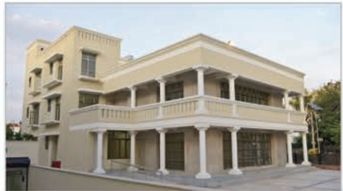
Banquet/ Community Centre, East Kidwai Nagar, New Delhi
