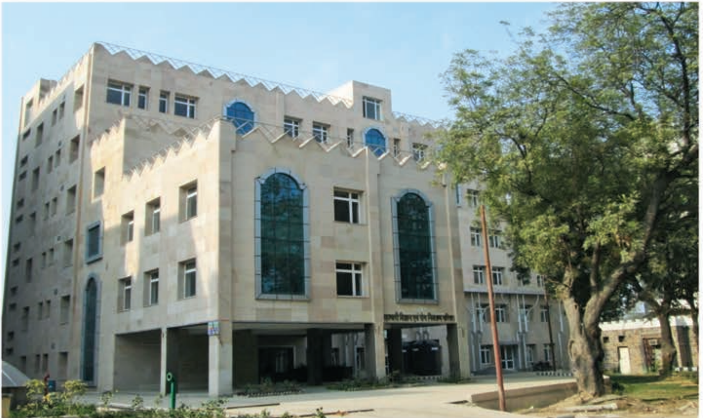
Dry Lab Building of National Centre for Disease Control (NCDC), Delhi
