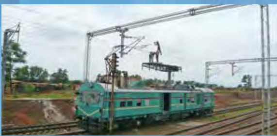
OHE job is in Progress.
