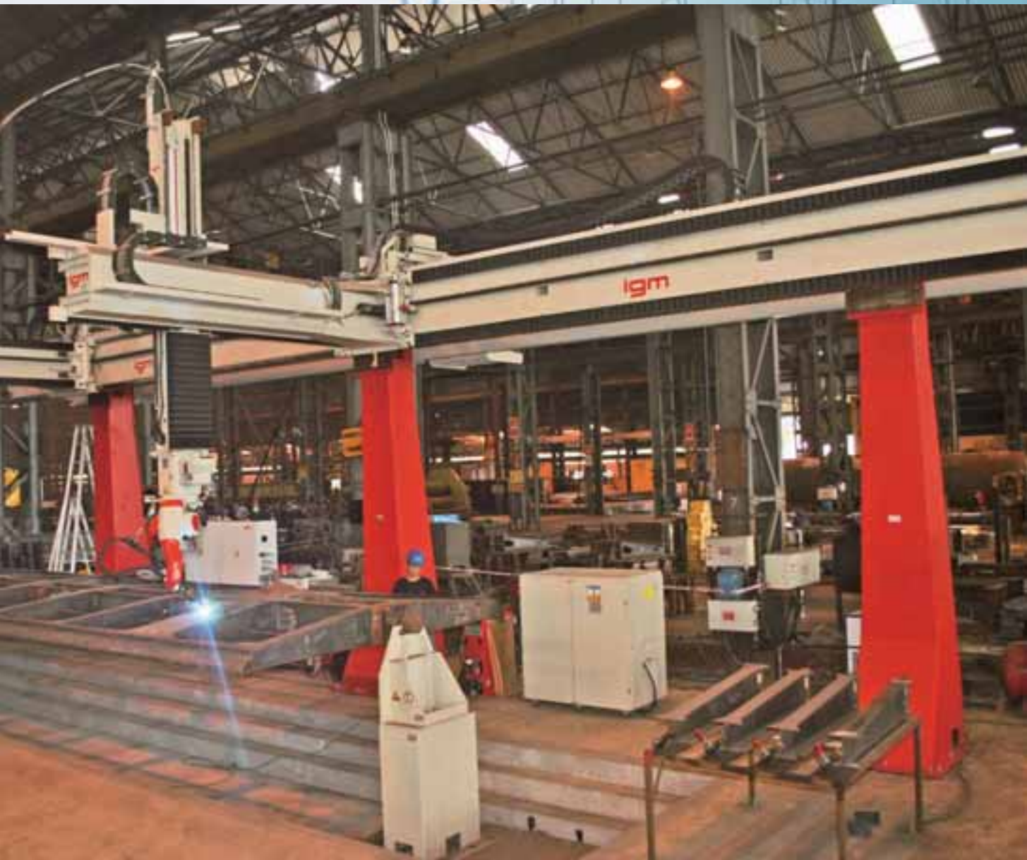
Robotic Welding Machine (IGM) at Agarpara Shop (under commissioning)
