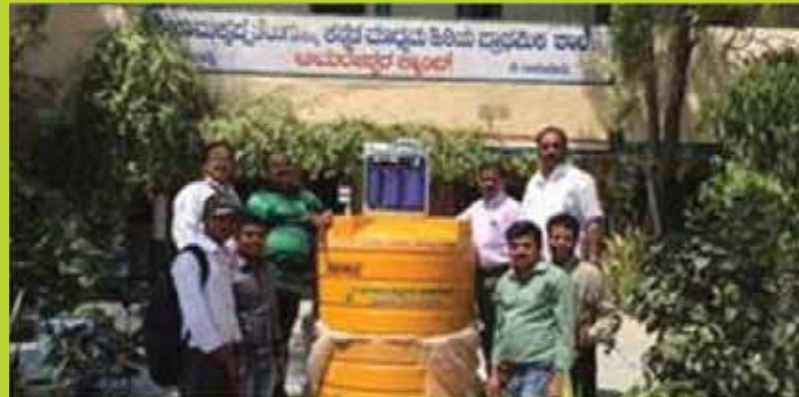
Installation of Water Storage Tanks in Bellary, Karnataka
