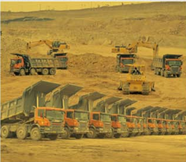
Rohtak-Panipat Section of NH-17a : work in progress
