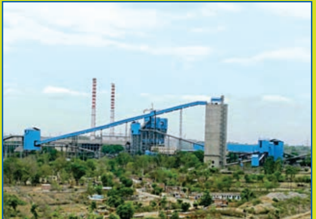
Captive Power Plant, Churk (U.P.)
