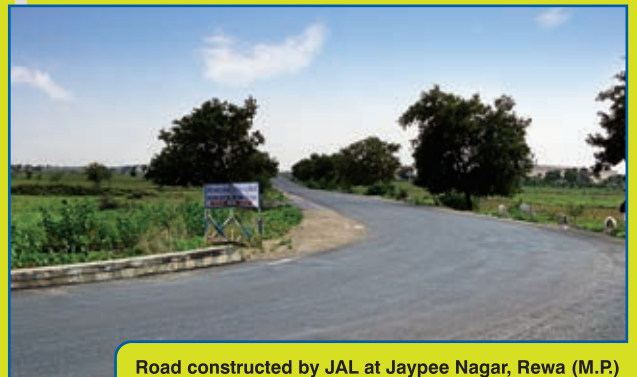
Road constructed by JAL at Jaypee Nagar, Rewa (M.P.)
