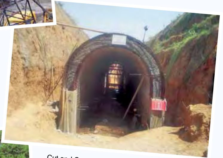
Cut and Cover - NW Railway Tunnel Lalsot, Jaipur (Rajasthan)
