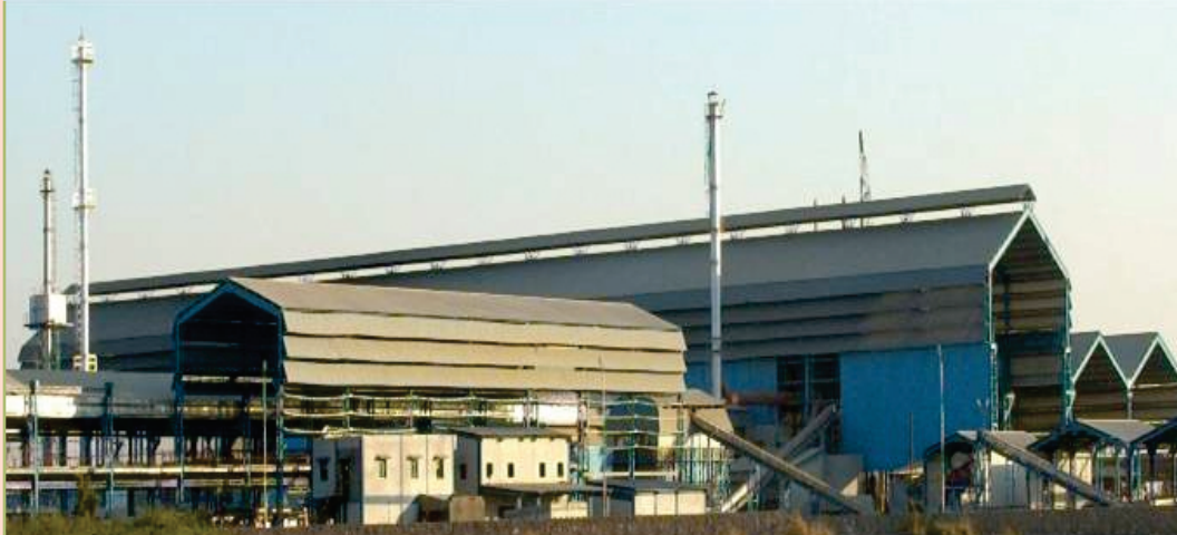
Plant at Samakhiali, Kutch
