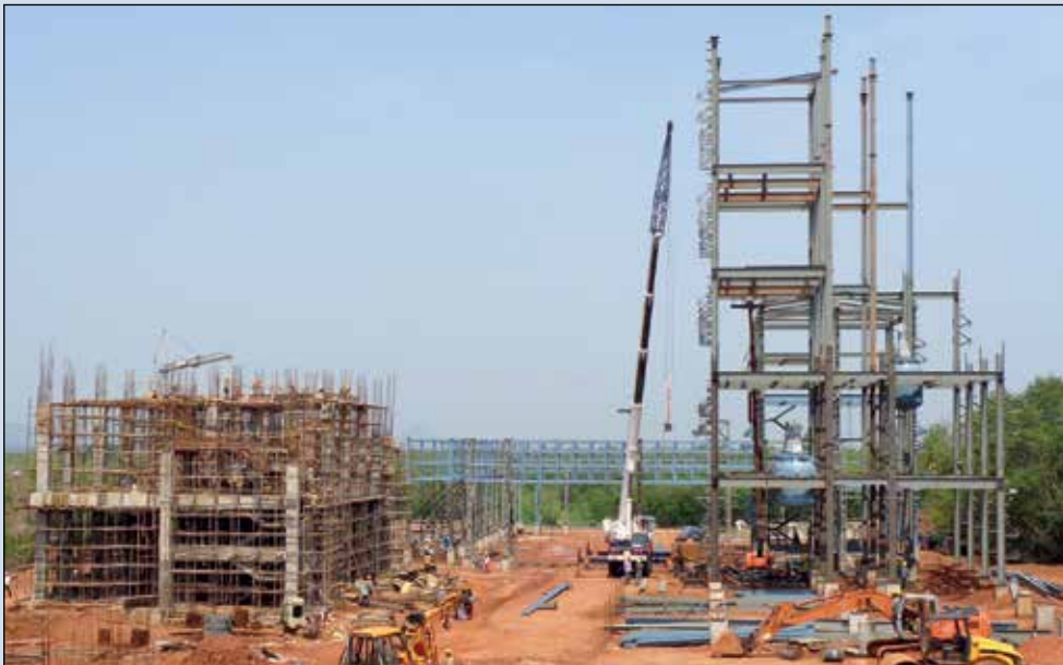
NACL Srikulam Tehcnical Unit - Block 7 implementation in progress
