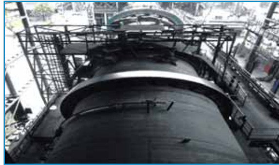
Kiln1 after renovation
