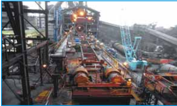
Kiln 1 in Dismantled Condition
