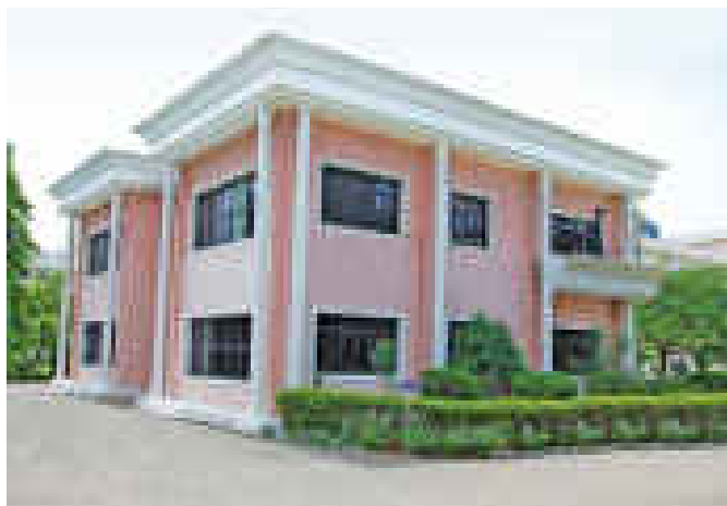
State-of-the-art US FDA approved API facility at Panoli, Gujarat
