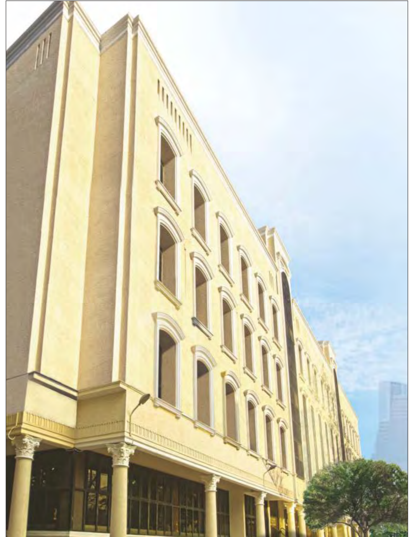
Actual Photograph - Elevation
