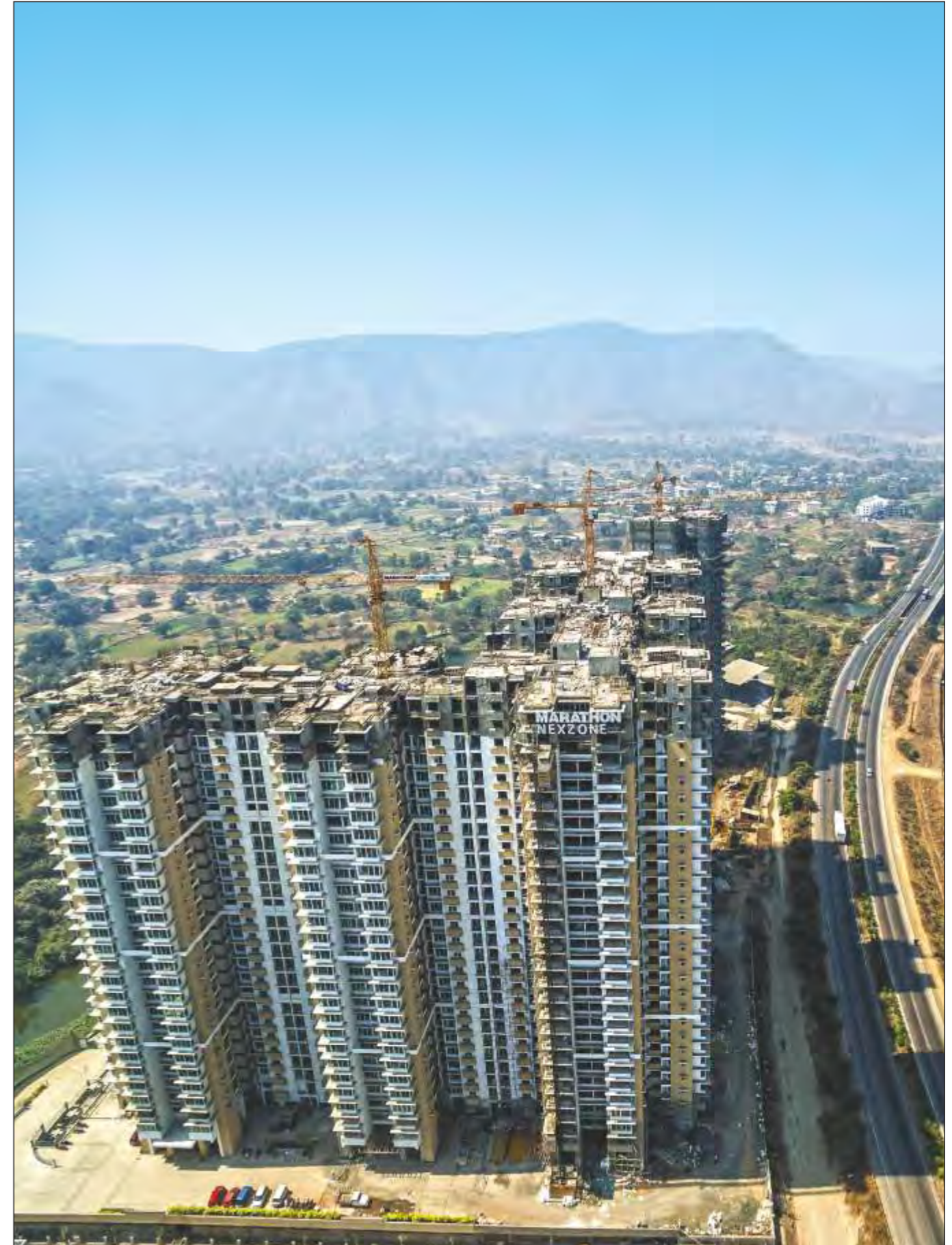
Actual Image - Construction status at Marathon Nexzone
