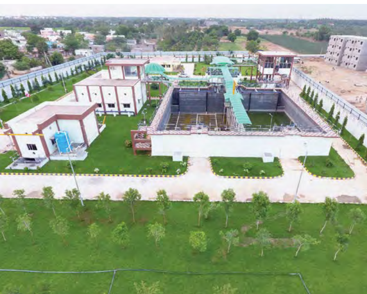
5 MLD Sewage Treatment Plant, Nellore
