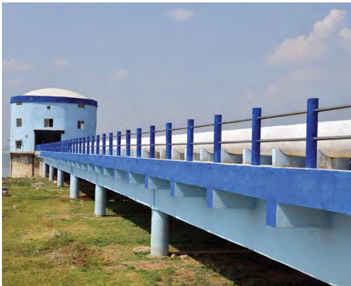
Medak and Sangareddy Water Supply Project
