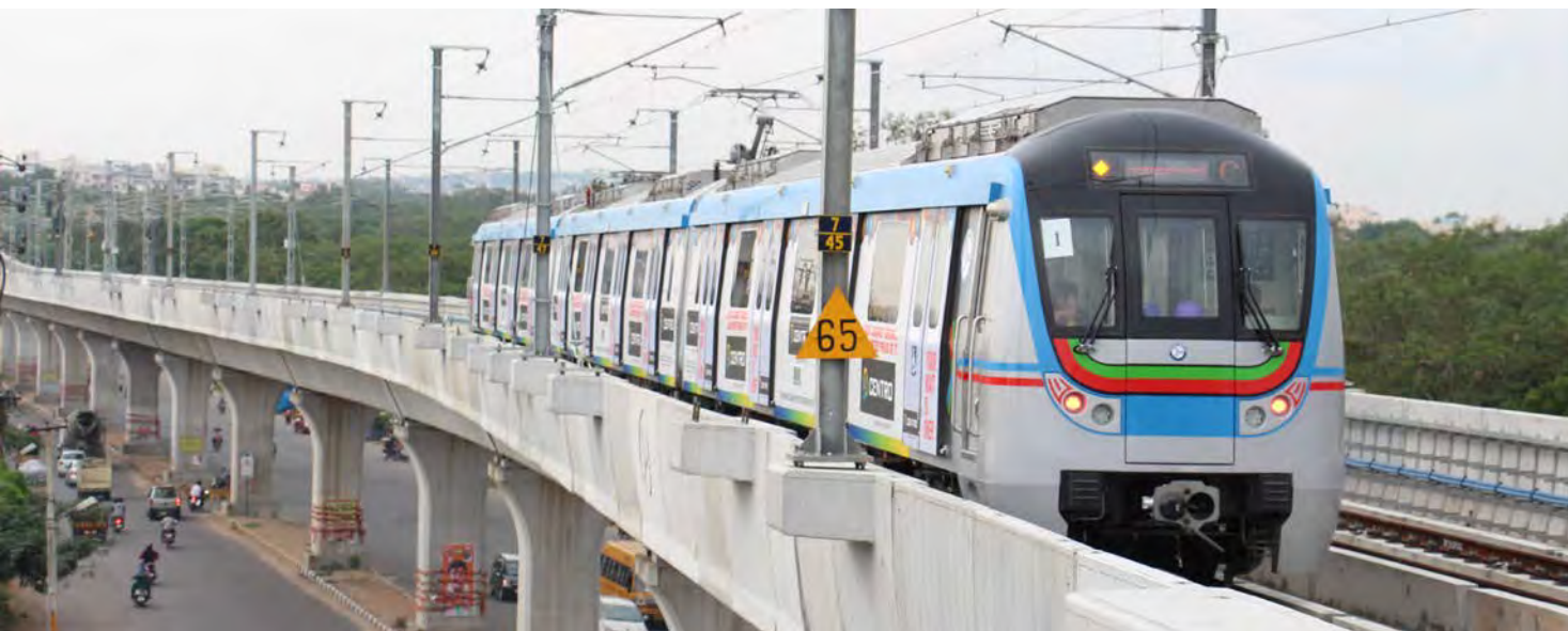
A section of the Hyderabad Metro
