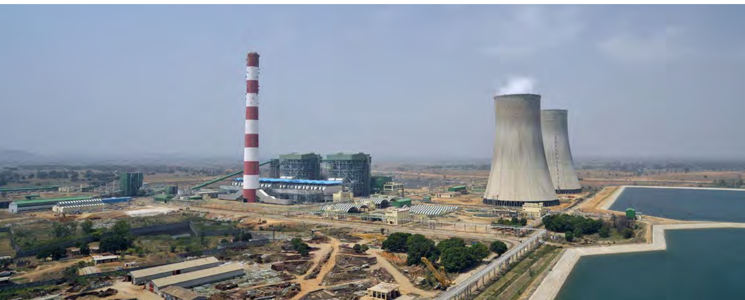
2x660 MW Jaypee Nigrie Thermal Power Plant, Madhya Pradesh
