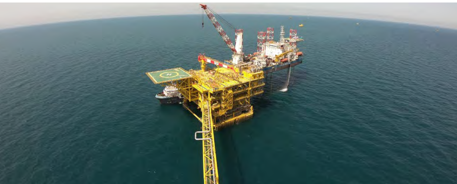
A fully-integrated gas platform - the heaviest in Saudi Aramco's history - installed by float-over method at Hasbah Field in Saudi Arabia
