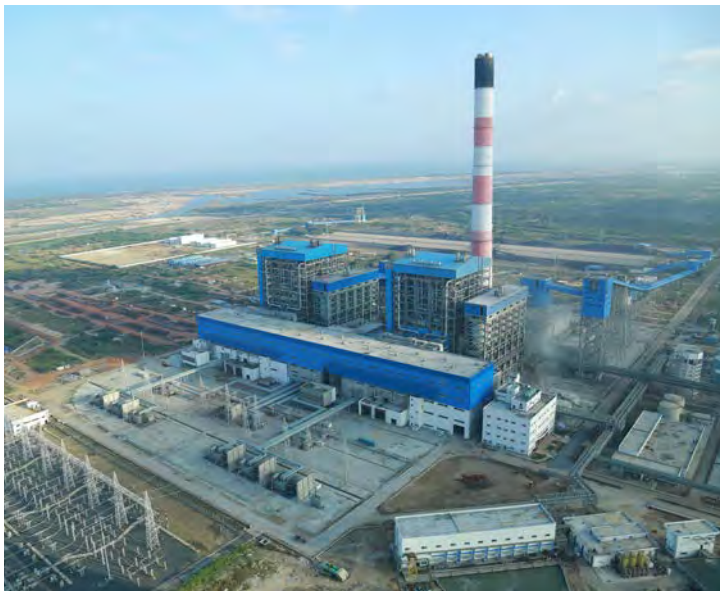
2x800 MW Sri Damodaram Sanjeevaiah Thermal Power Plant, Andhra Pradesh
