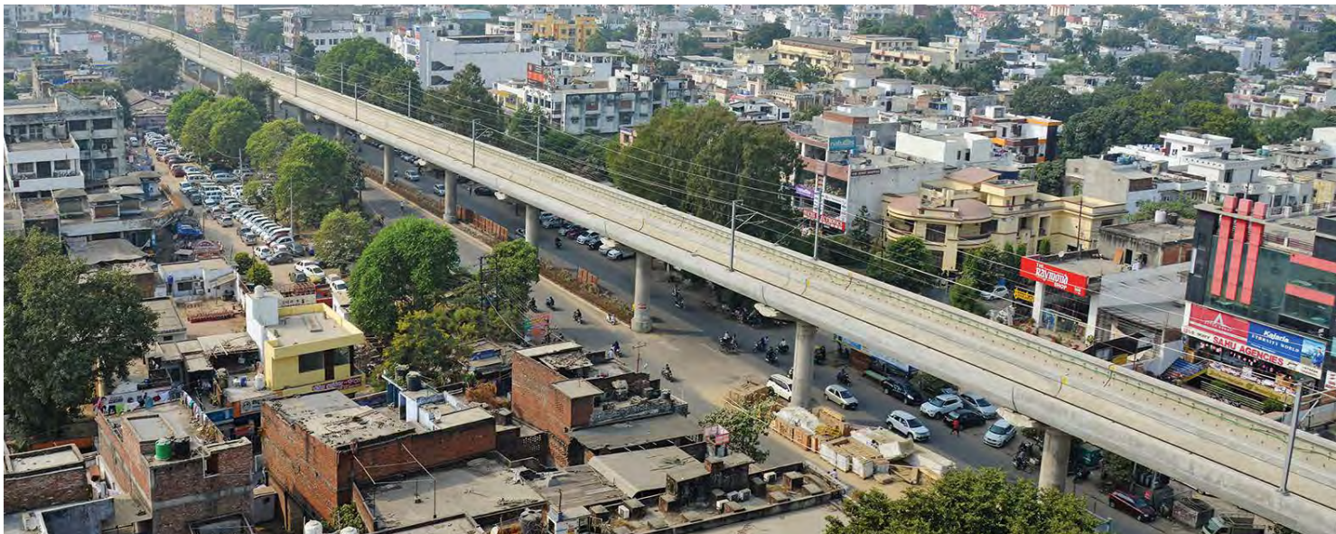
Lucknow Metro - one of the fastest completed metro projects in India
