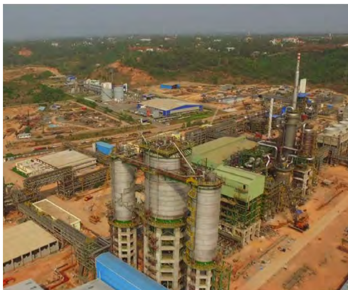
Panoram view of PTA Plant for JBF Industries, Mangalore
