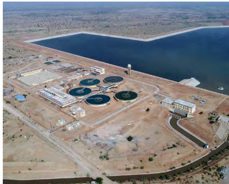
Overview of Nagaur 250 MLD Water Treatment Plant and 5310 ML Raw Water Reservoir
