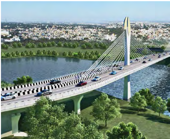
Cable-stayed bridge across Durgam Cheruvu Lake, Telangana
