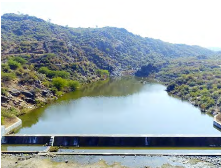
L&T has built over 200 check dams in water stressed areas
