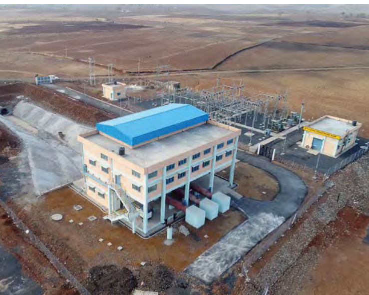
Pump house for Mohanpura Lift Irrigation Scheme
