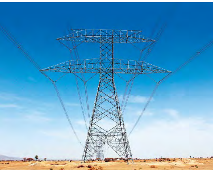
400 kV Ibri-Izki Transmission Line, Oman
