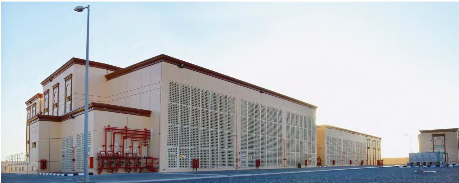
132/33/11kV Substation, Umm Al Quawain, UAE
