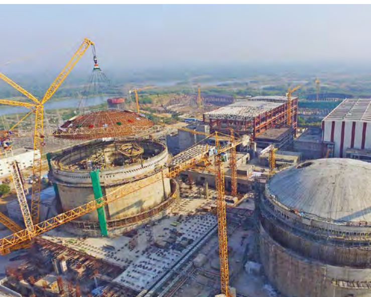
Kakrapar Atomic Power Plant, Gujarat, under construction
