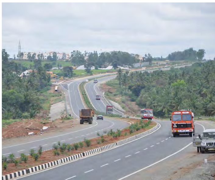
Devihalli Hassan Toll Road
