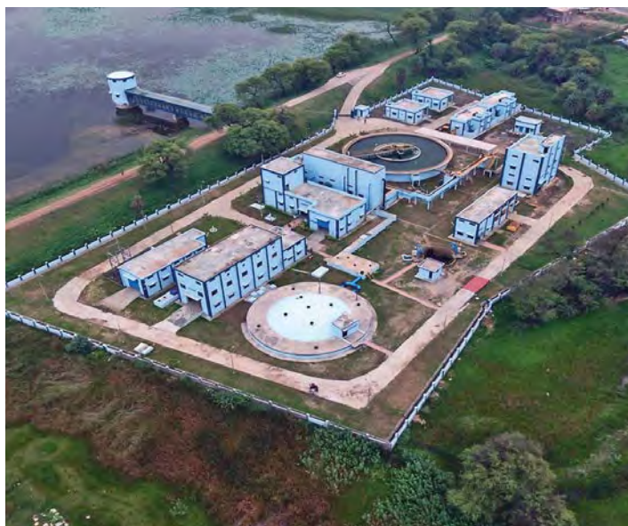
10.6 MLD Water Treatment Plant, Bagidora
