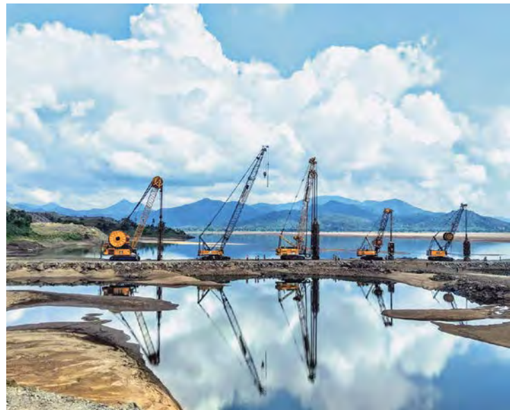
Cut-off-wall, Polavaram Dam, Andhra Pradesh
