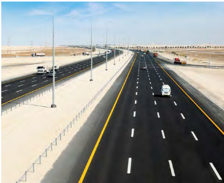
Mafrag-Ghweifat Highway, Abu Dhabi
