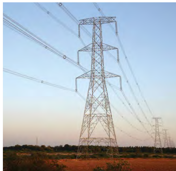
765 kV DC Kudgi Transmission Line project
