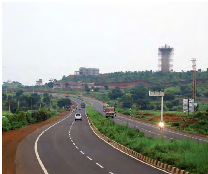
Solapur-Sangareddy Road Project
