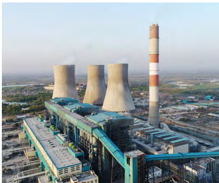
3x660 MW Koradi Thermal Power Plant, Maharashtra
