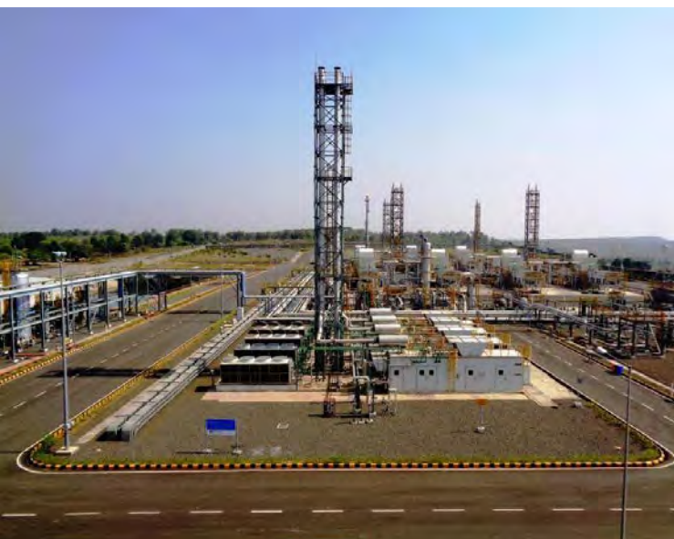
Group Gathering Station-11 for RIL's Coal Bed Methane Field Development Project, Shahdol, Madhya Pradesh
