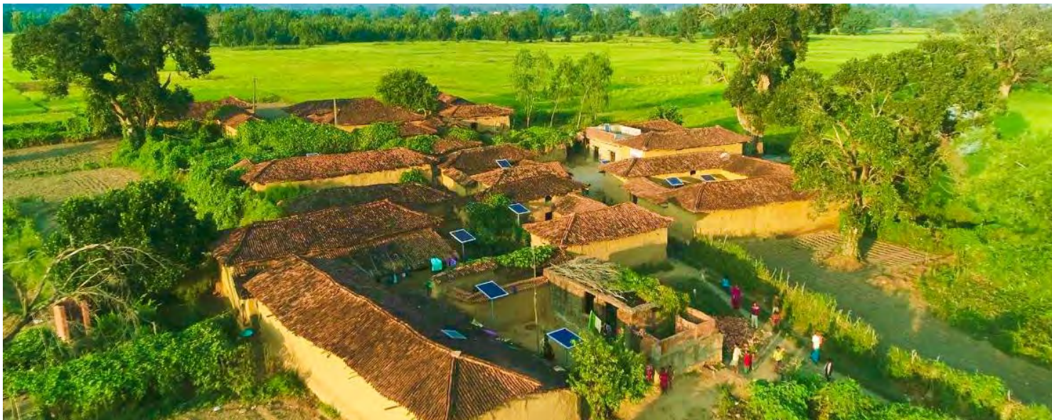
Micro Grid Project for rural electrification, Bihar
