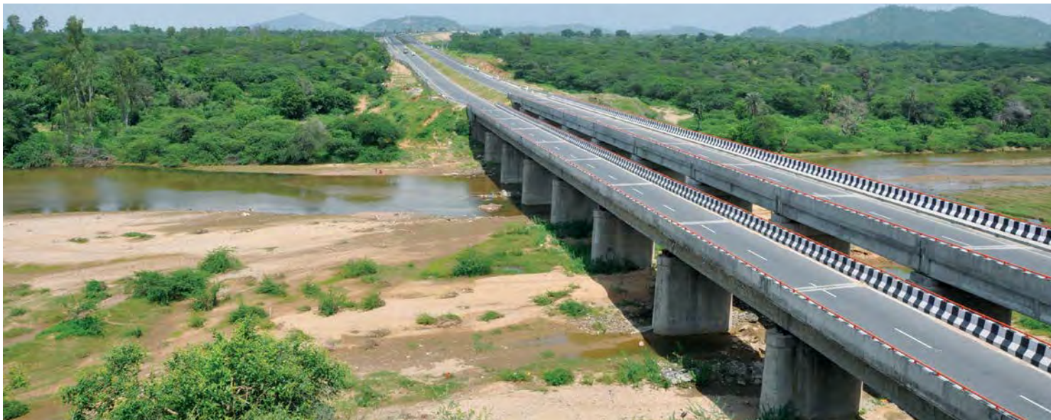
NH-14 Palanpur-Swaroopganj Highway
