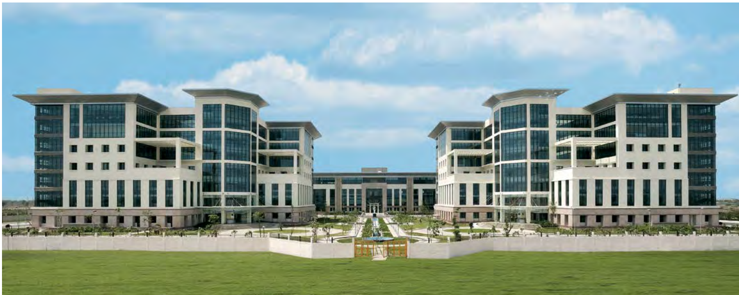
Headquartered at Knowledge City, Vadodra, L&T Technology Services helps clients gain the competitive edge by building smart products, enabling smart manufacturing and offering smart services.
