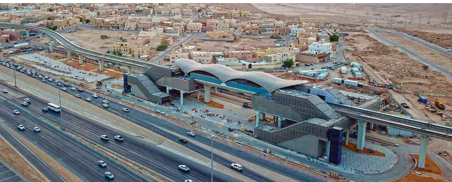
Riyadh Metro - L&T is building metro networks in India and select geographies
