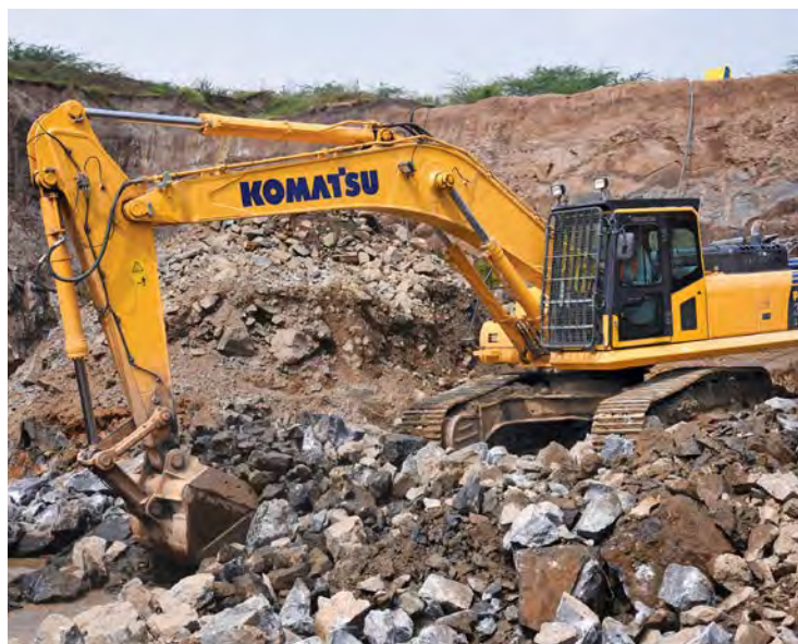
Komatsu PC350LC-8M0 Hydraulic Excavator
