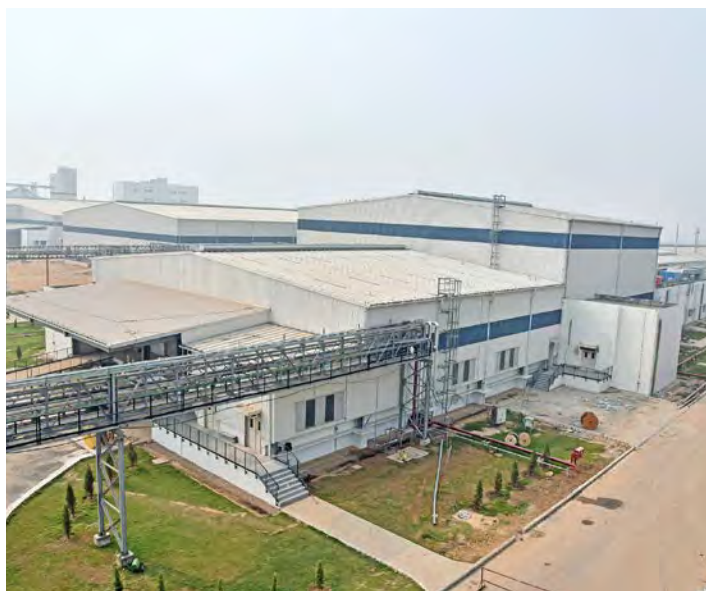
ITC Food Manufacturing and Logistics Facility, Kapurthala
