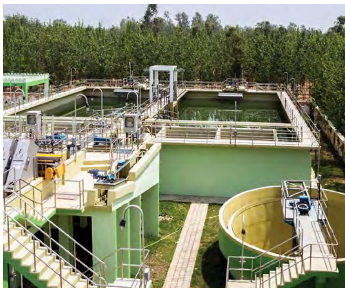
Sewage Treatment Plant at Rampur
