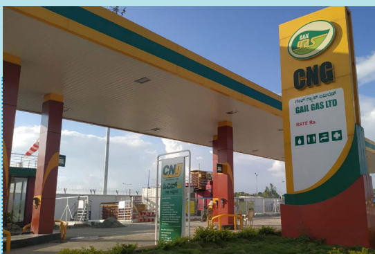
City Gas Distribution (CGD) Projects
