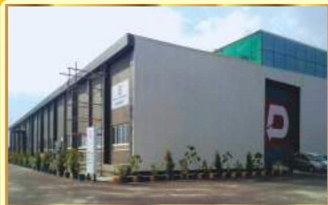
Deffence Manufacturing unit at Devanahalli - Bangalore
