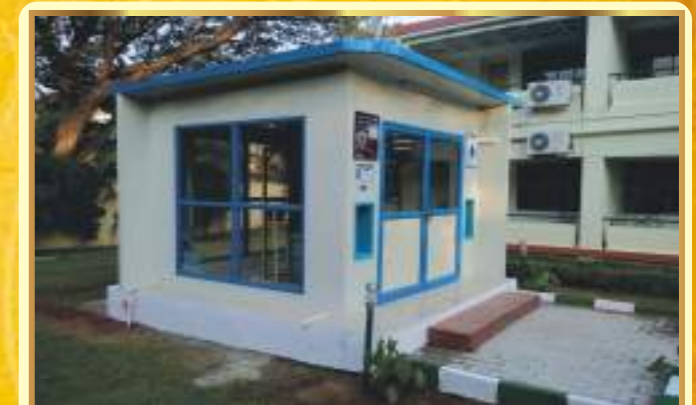
R.O Water Plant at Mysore- Completed 2000 No's in Karnataka
