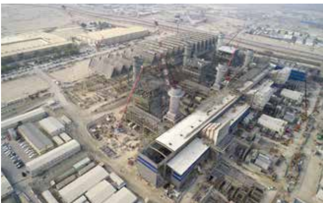
Alba PS51800 MW CCPP Project, Kingdom of Bahrain
