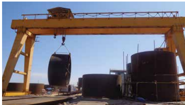
2 x 700 MW, RAPP, Rajasthan
