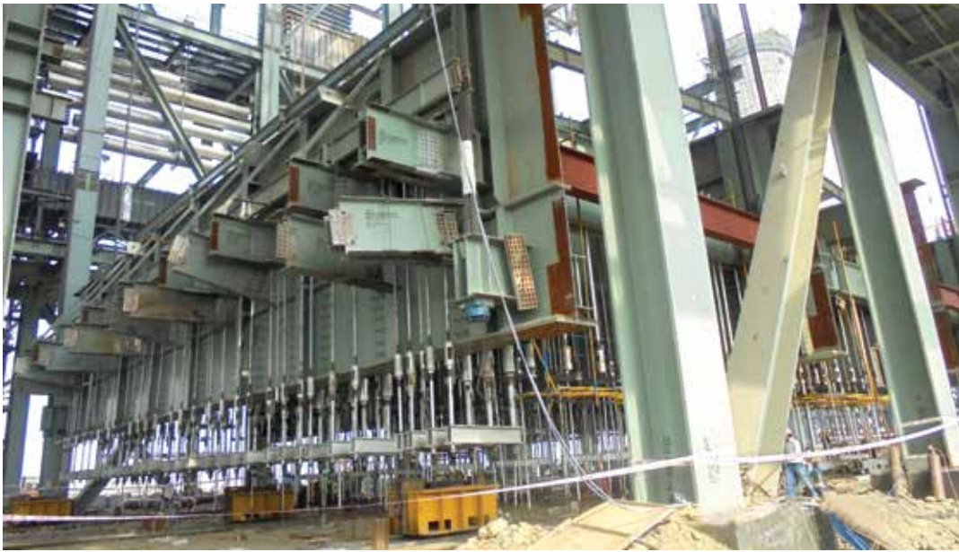
2 x 660 MW Chhabra TPP, Lifting Ceiling Girder 3030 MT
