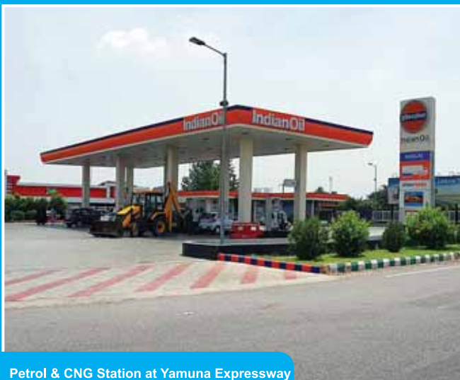
Petrol & CNG Station at Yamuna Expressway
