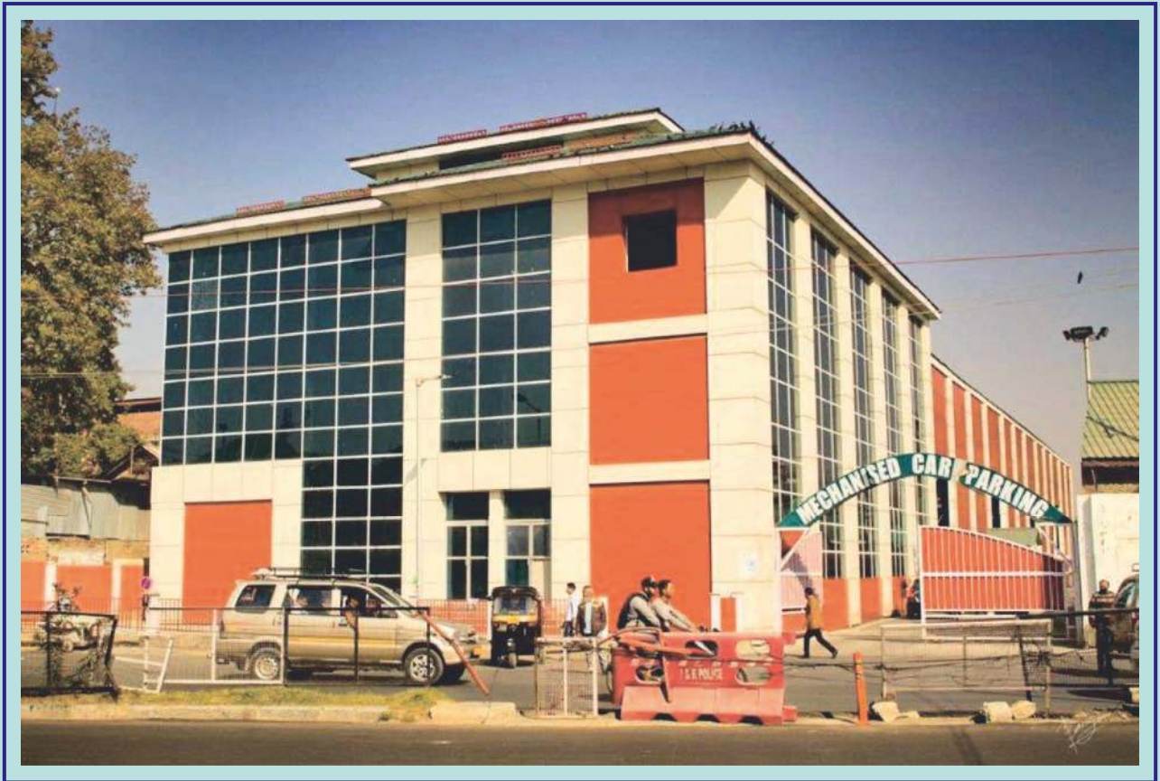
MECHANISED CAR PARKING, Srinagar
