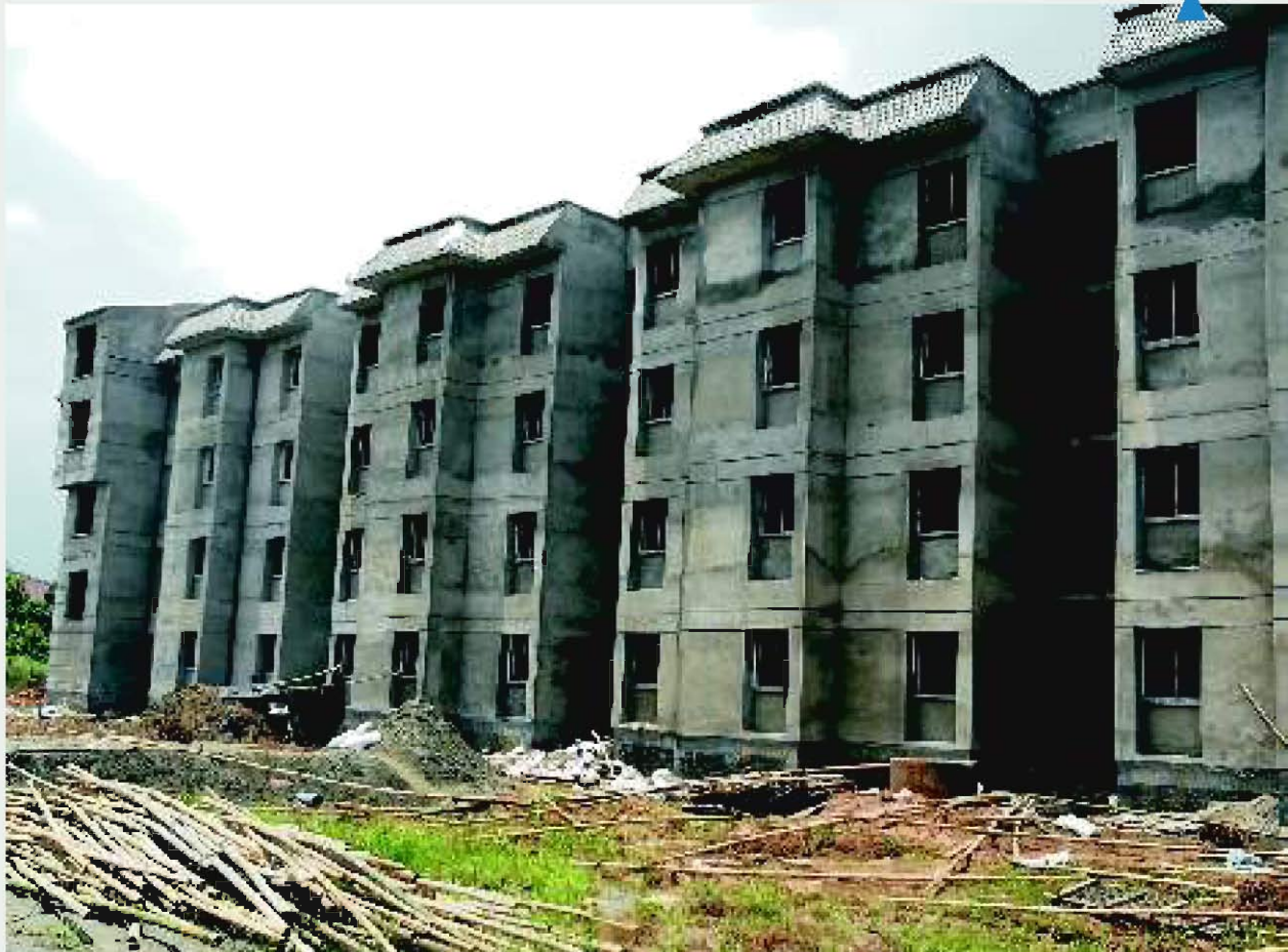
Boys Hostel at IIT Guwahati Campus (under construction)
