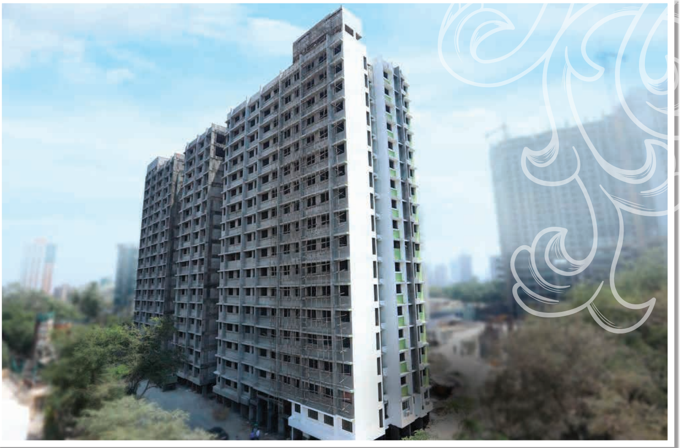
(Original Construction Project Photo)
