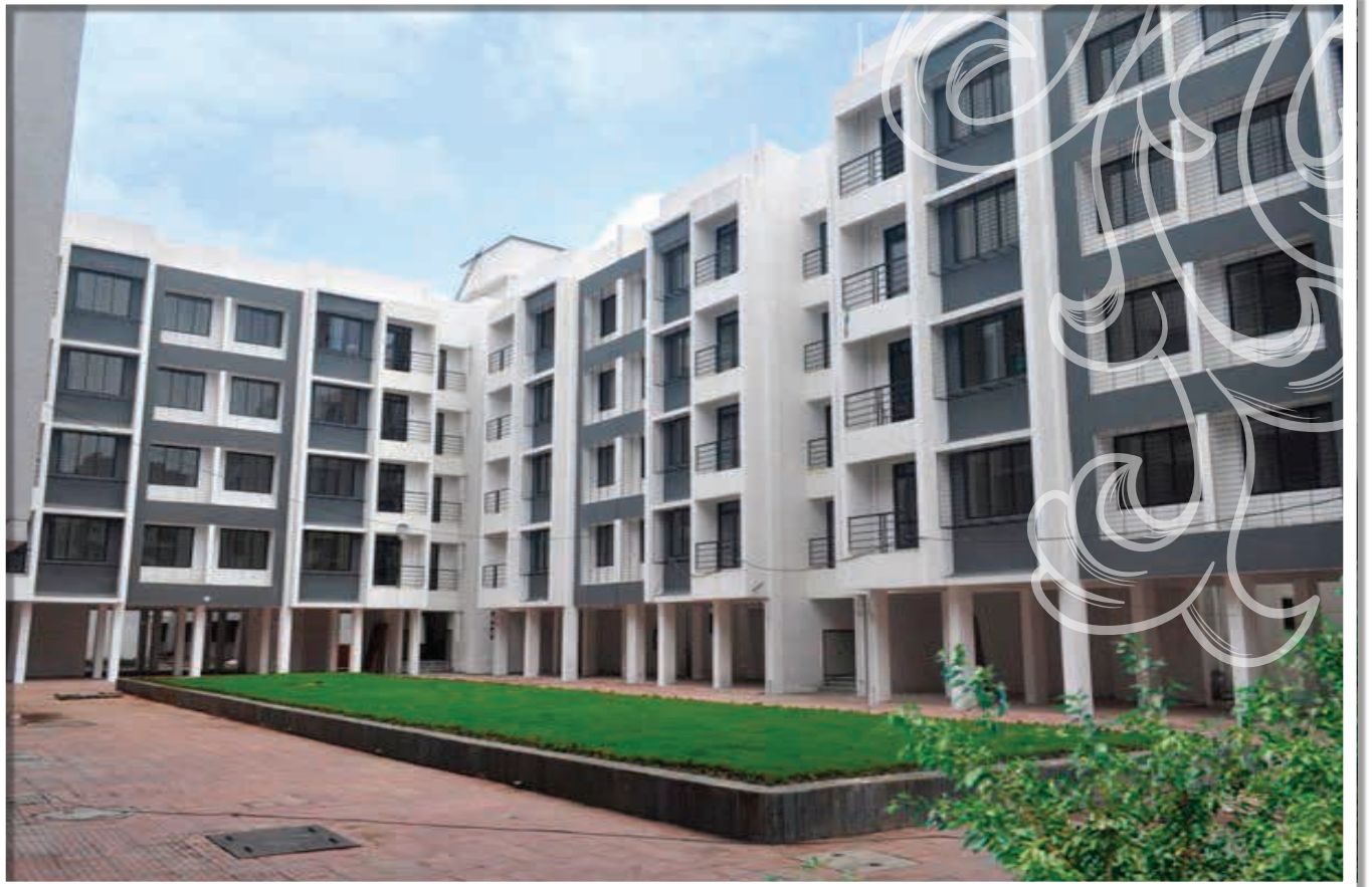
(Original Construction Project Photo)
