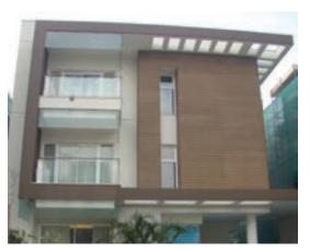
noise absorbent and also has fire resistant properties. The alkali resistant glass fibres used in GFRC contain high percentage of Zirconium, which increases the flexural strength of concrete. Customized products can be made with GFRC which can be easily installed at site and requires low maintenance.
