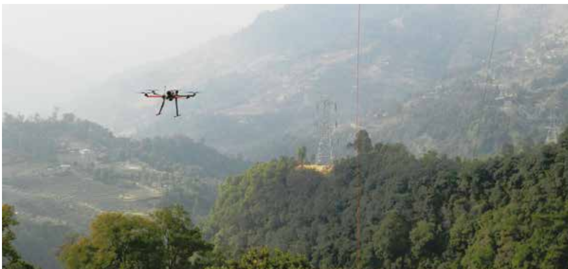
Stringing of power conductors using drone, Bhutan
