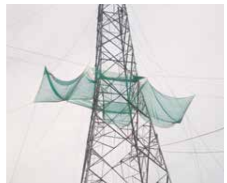
Safety Net to reduce the impact of fall
