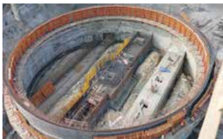
Specialised Climbing Formwork technology for construction of heavy silo structures
