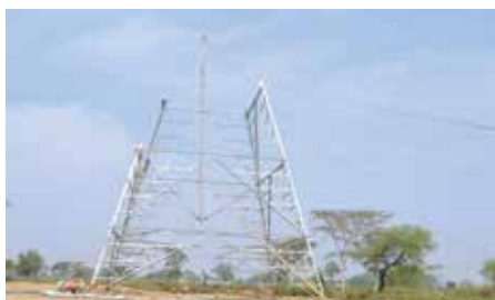
Deployment of Gin Poles for tower erection at 765 kV Raigarh – Pugalur Transmission Line
