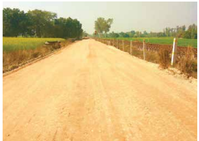
Blanketing work for track-laying at Amethi, Uttar Pradesh
