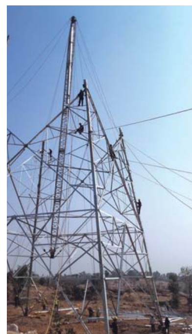
► Use of Gin Poles for Tower Erection
