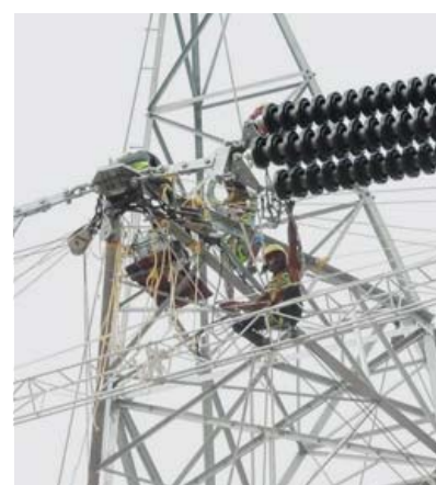
► Stringing using Sag Bridges
