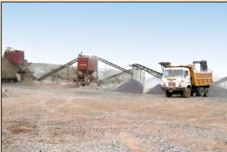
150 TPH 3 STAGE STONE CRUSHING UNIT
