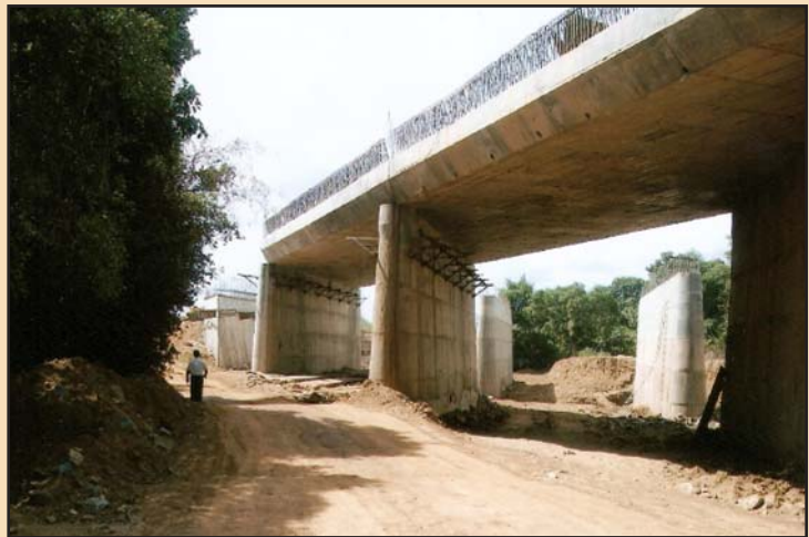
45° SKEW BRIDGE CONSTRUCTION AT SAWANTWADI
