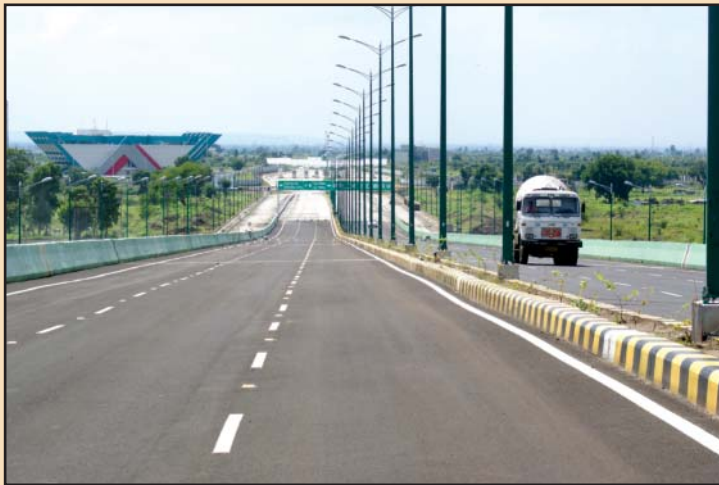
6 LANE ROAD CONSTRUCTED FOR MIHAN SEZ, NAGPUR
