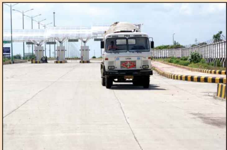
6 LANE CONCRETE PAVEMENT FOR MIHAN SEZ, NAGPUR
