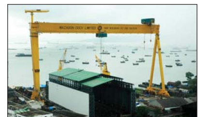
300Tons Goliath crane.Mazagon Docks
