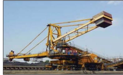
Stacker Reclaimer.Satpura TPP
