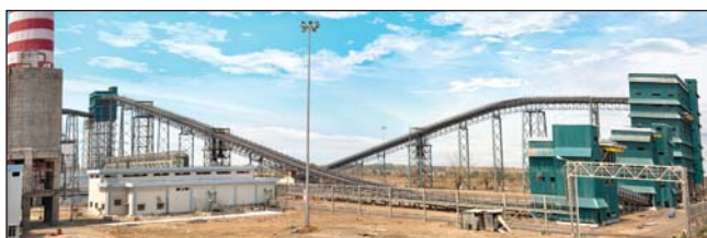
Coal Handling Plant, Ideal Power
