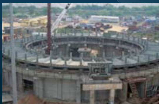
Circular Sinter Cooler (under construction)
