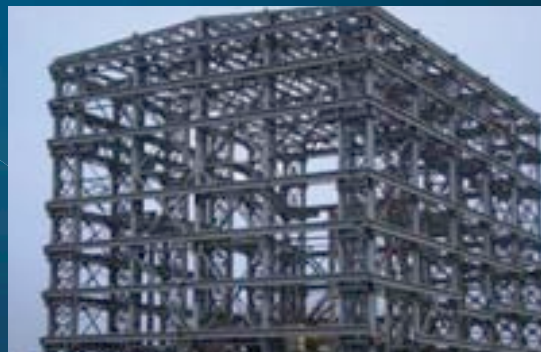
By Products plant, IISCO, Fabricated structure
