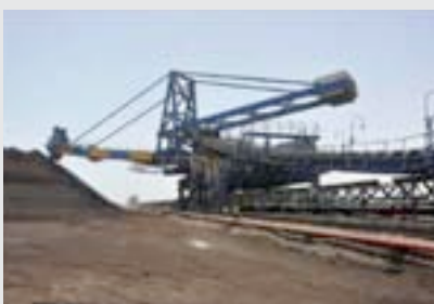
Stacker Reclaimer, Adani Port
