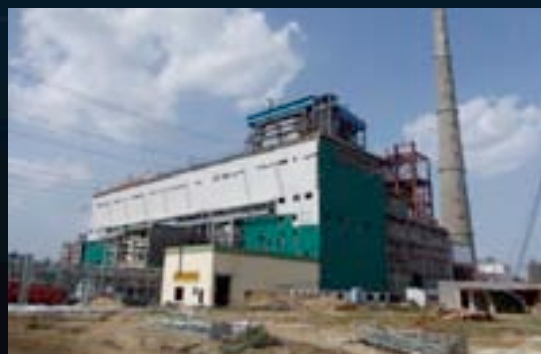
Ideal Power Plant (under construction)
