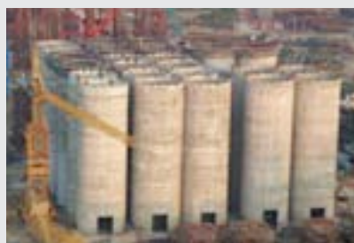
Coal Silos under construction, SAIL Rourkela
