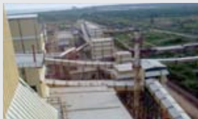
Aerial view, Sinter Plant, Vizag Steel
