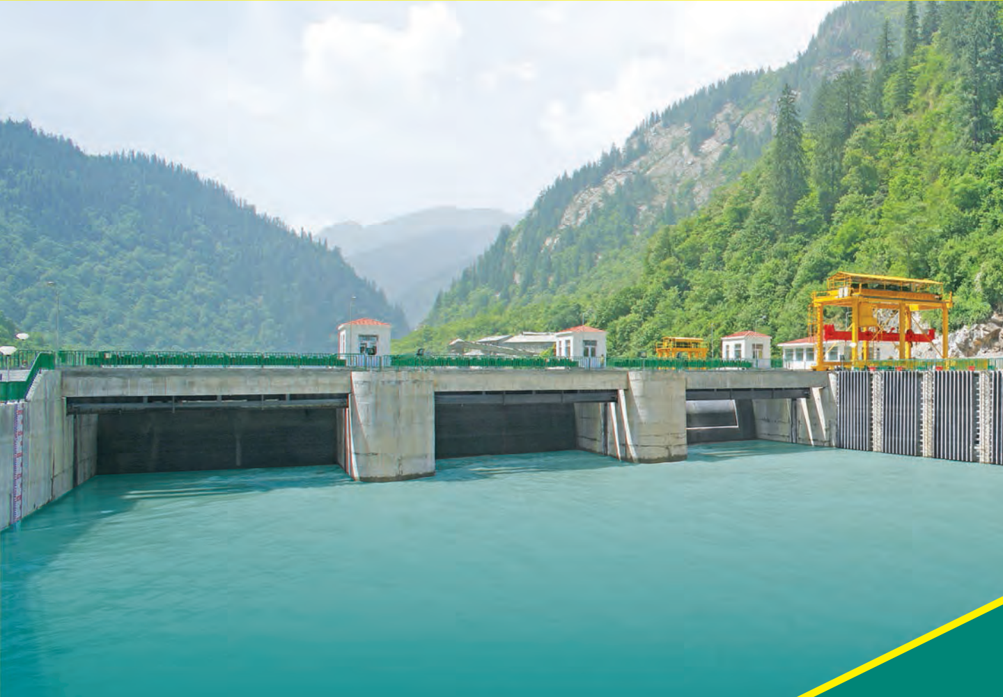
Upstream View of 400 MW Vishnuprayag Barrage, Uttarakhand
