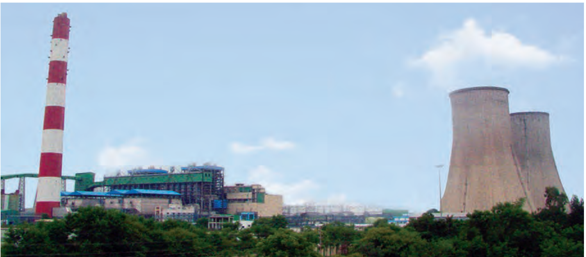
500 MW Bina Thermal Power Plant, Bina, Madhya Pradesh
