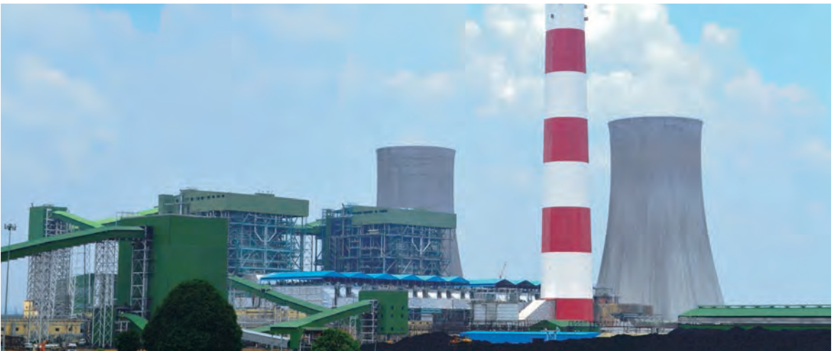
1320 MW Jaypee Nigrie Super Thermal Power Plant, Nigrie, Madhya Pradesh
