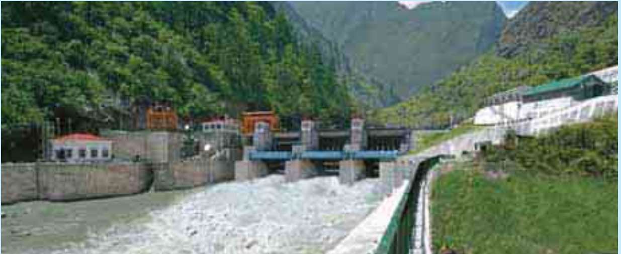
400 MW Vishnuprayag Dam, Uttarakhand (In Operation)
