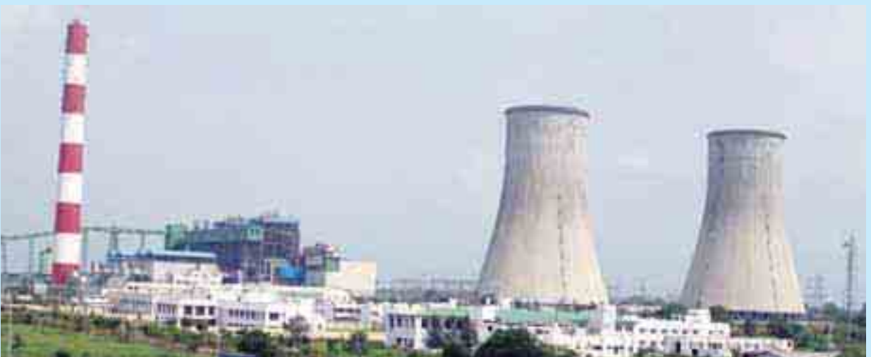
500 MW Bina Thermal Power Plant, Bina, Madhya Pradesh (In Operation)
