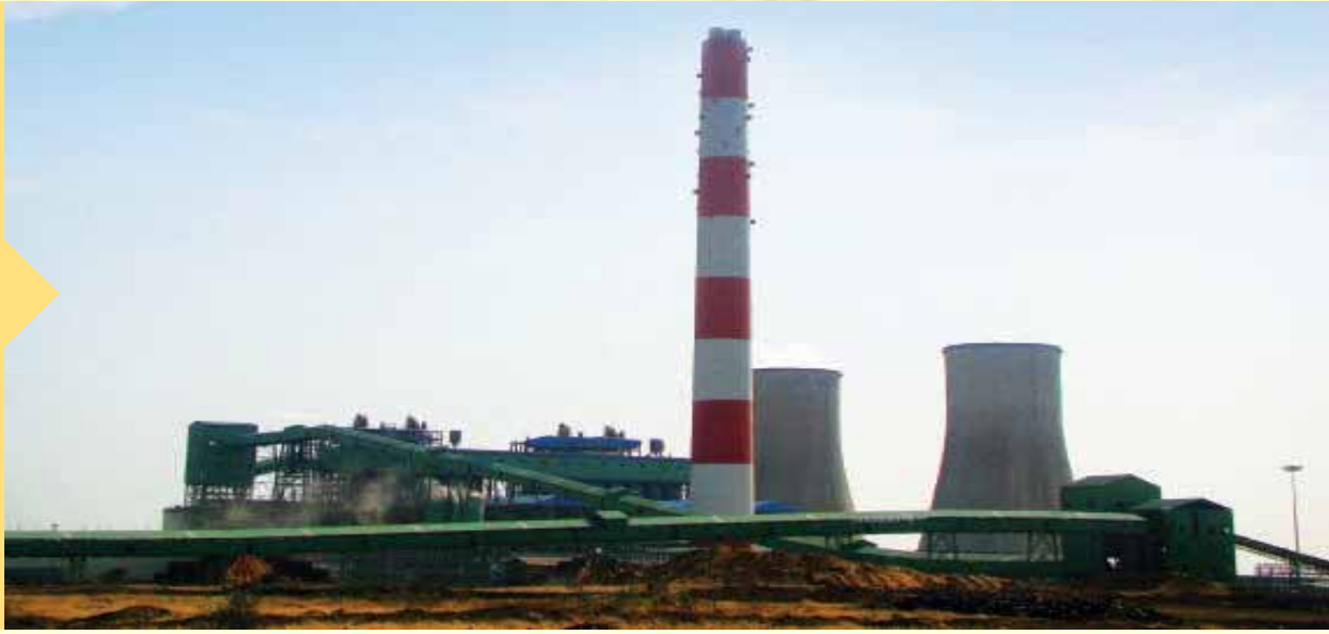
View of 500 MW Bina TPP (Phase-I) Madhya Pradesh
