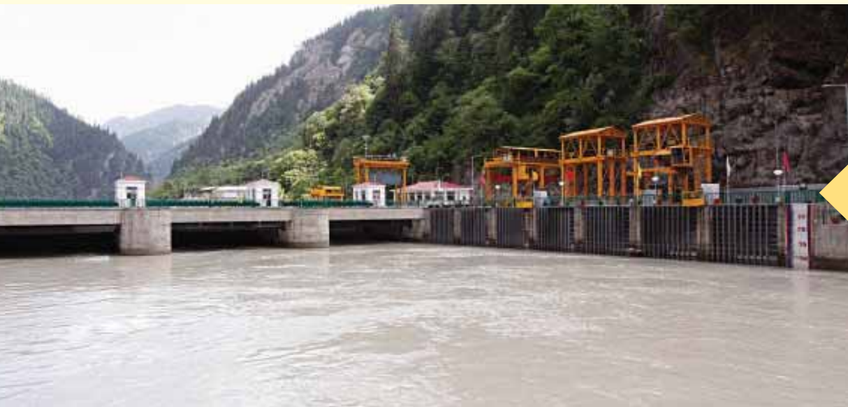
Upstream view of Barrage of 400 MW Vishnuprayag Hydro Electric Plant, Uttarakhand
