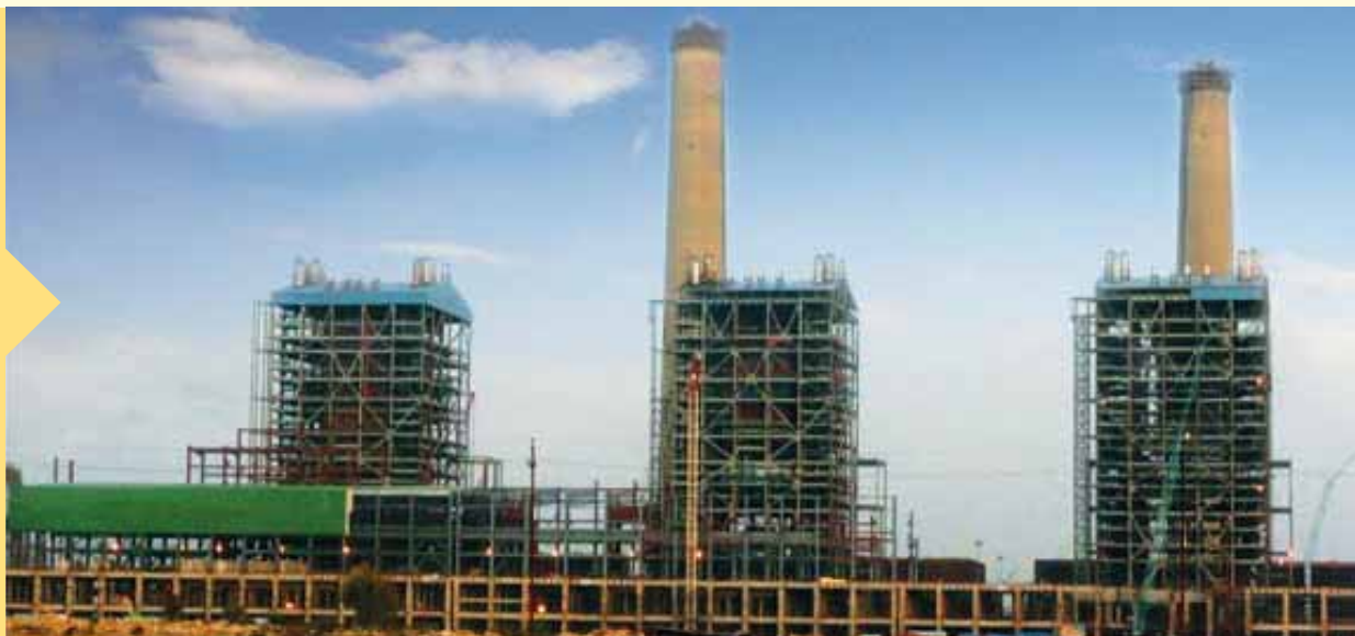
Work in progress at 1980 MW Bara Supercritical TPP (Phase-I) Uttar Pradesh
