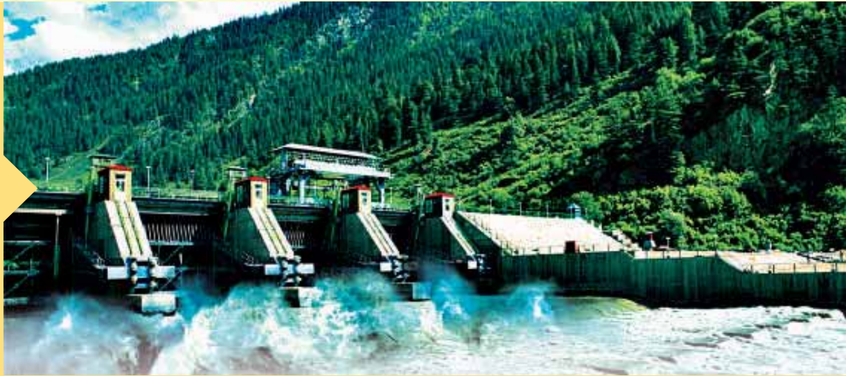
Barrage of 300 MW Baspa-II Hydro Electric Plant, Himachal Pradesh
