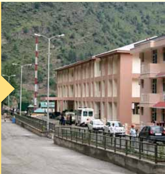
40 bed hospital at Sholtu, Himachal Pradesh
