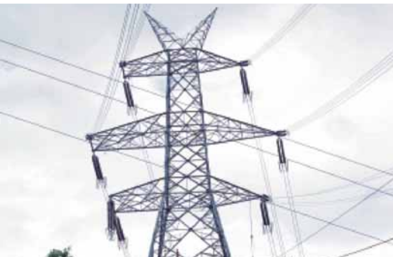
Transmission line of Jaypee Powergrid from Wangtoo to Abdullapur
