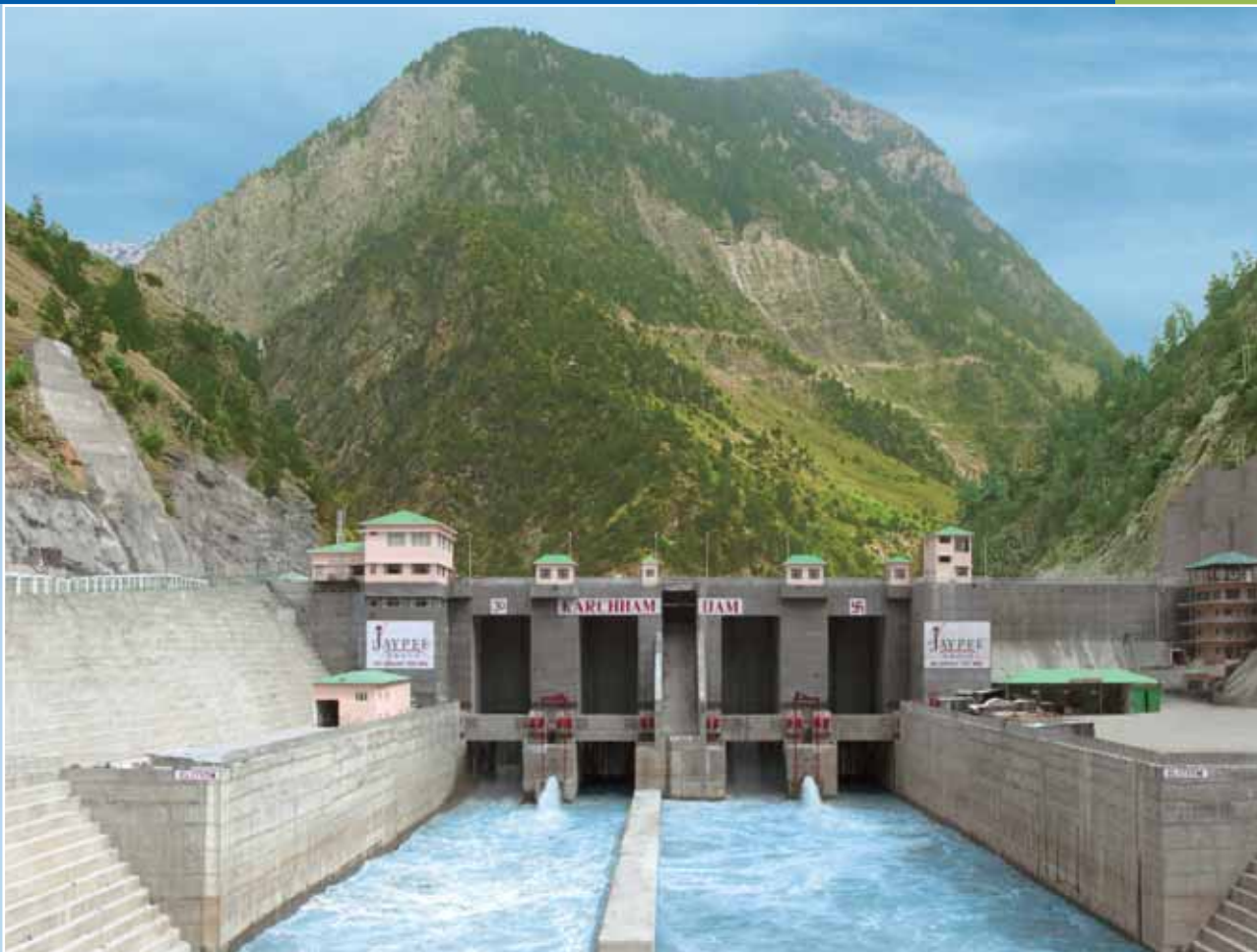
1000 MW Karcham Dam on River Satluj, H.P.
