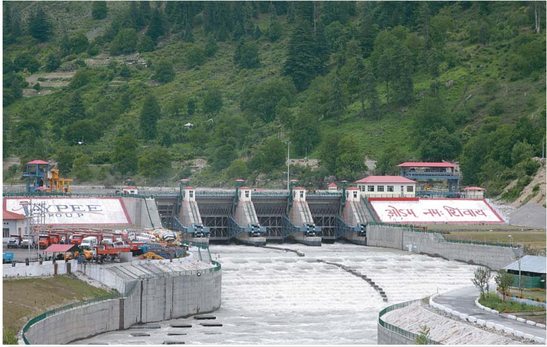
Barrage of 300 MW Baspa-II Hydro Power Station, Himachal Pradesh
