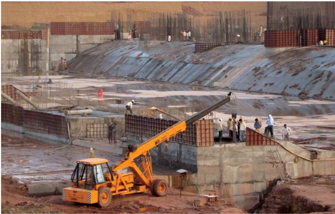
Barrage Under Construction at 500 MW Bina TPP (Phase-I) Madhya Pradesh
